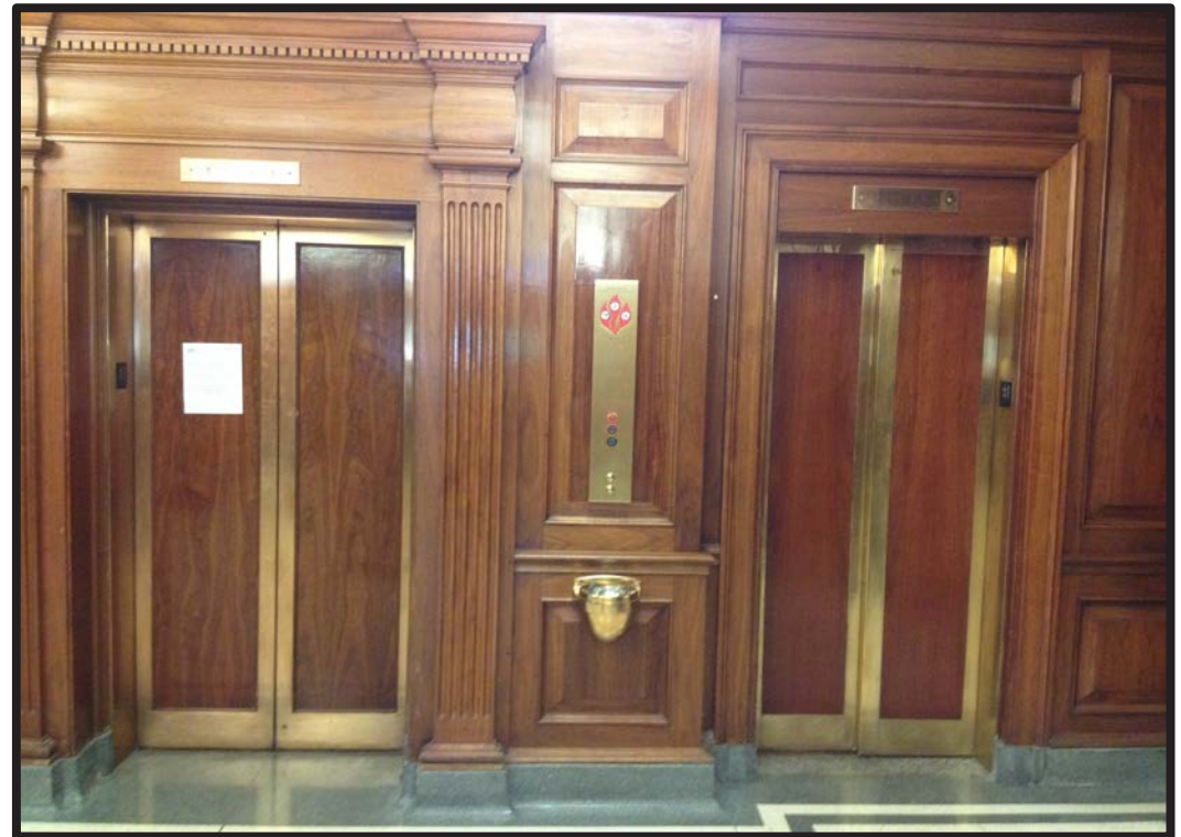
Project Location: Police Building at 10 S. Brentwood Ave 2015.PW.1404.410
