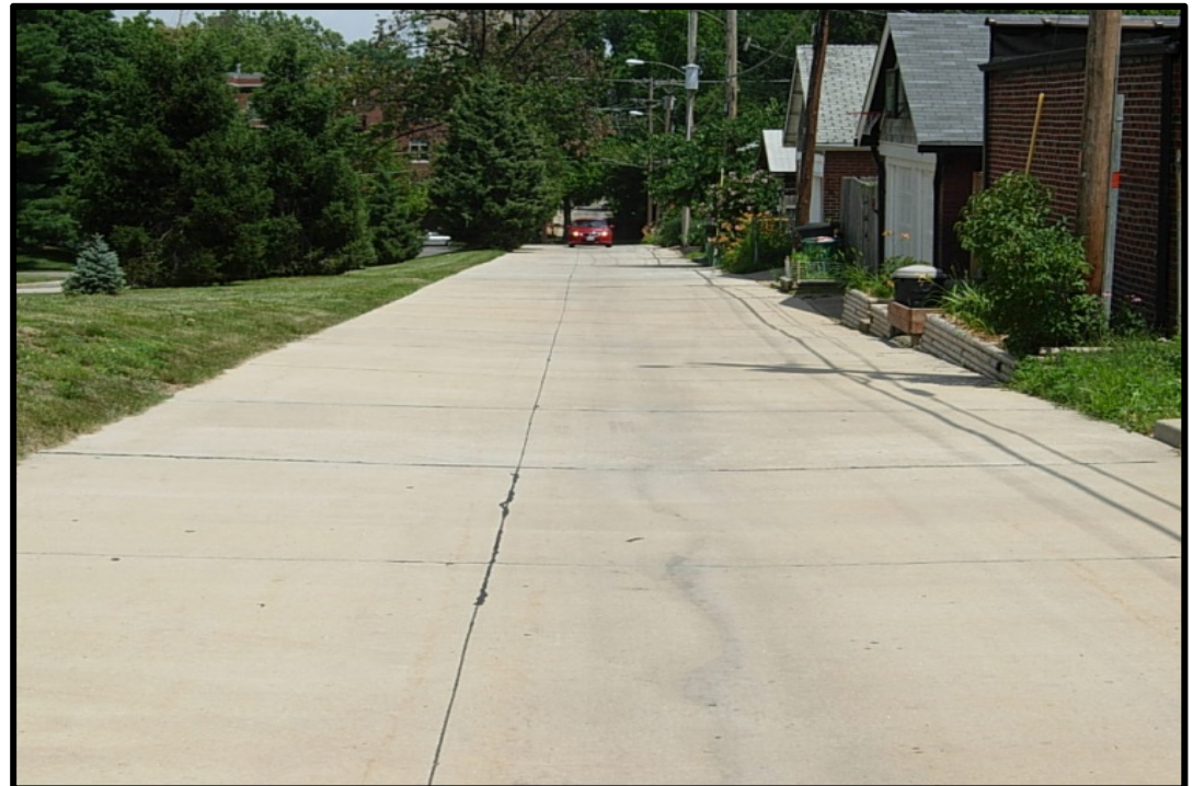
Project Location: Various Alleys 2014, 2015, and 2016.PW.1401.030 2015.PW.1401.031
