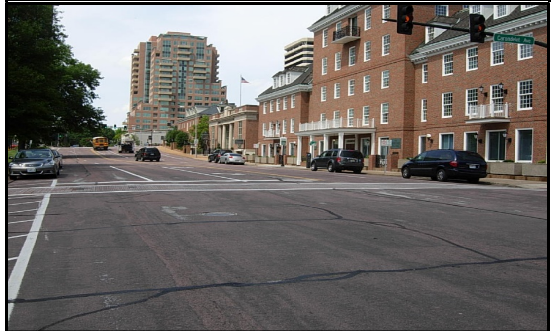
Project Location: Brentwood Blvd 2018.PW.1401.020
