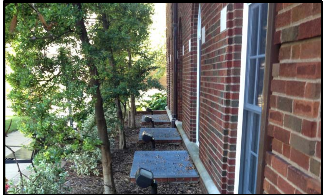
Project Location: 10 N. Bemiston Ave 2015.PW.1404.430 2013.PW.1404.420
