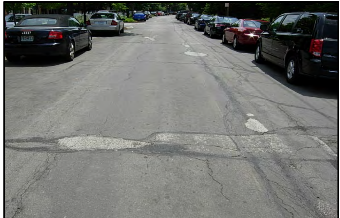
Project Location: Old Towne, Hanley Place, Skinker Heights, Hi Pointe, and DeMun Park Subdivisions 2014.PW.1401.010
