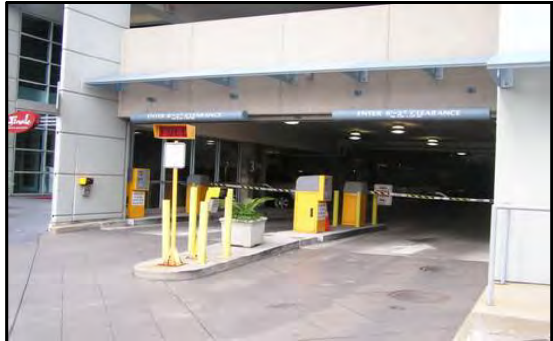
Project Location: 8011 Bonhomme Parking Structure 2014.PW.1406.600
