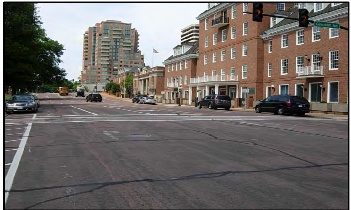
Project Location: Brentwood Blvd 2015.PW.1401.020
