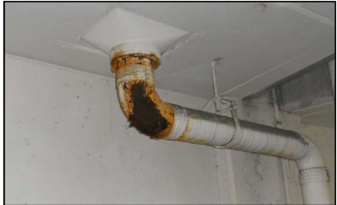
Project Location: 8011 Bonhomme Garage – All Stormwater Pipe 2013.PW.1404.450
