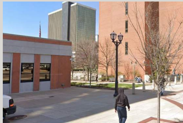
A building setback creates an open public space between the County Government Building and the County Courts allowing for community members and visitors to sit and enjoy a small open greenspace.
