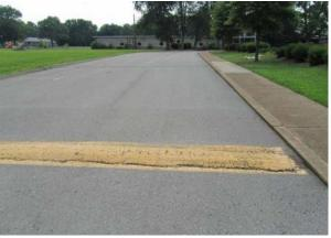
will be able to comfortably travel at the posted speed limit. In contrast, speed bumps require vehicles to travel much slower to attain a comfortable travel speed. Speed bumps can also lead to traffic using an alternate route which creates a problem at another location. Emergency service vehicles can experience delays and damage to equipment due to speed bumps. In summary, speed bumps should not be installed on public roads and are not considered to be a traffic calming measure.
