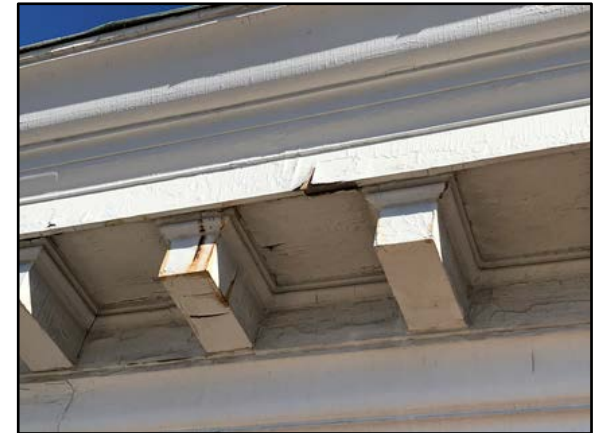
Project Location: 10 S. Brentwood Blvd 2021.PW.1404.440
