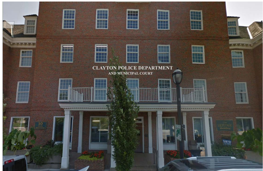
Project Location: 10 S. Brentwood Blvd 2020.PW.40.42.442
