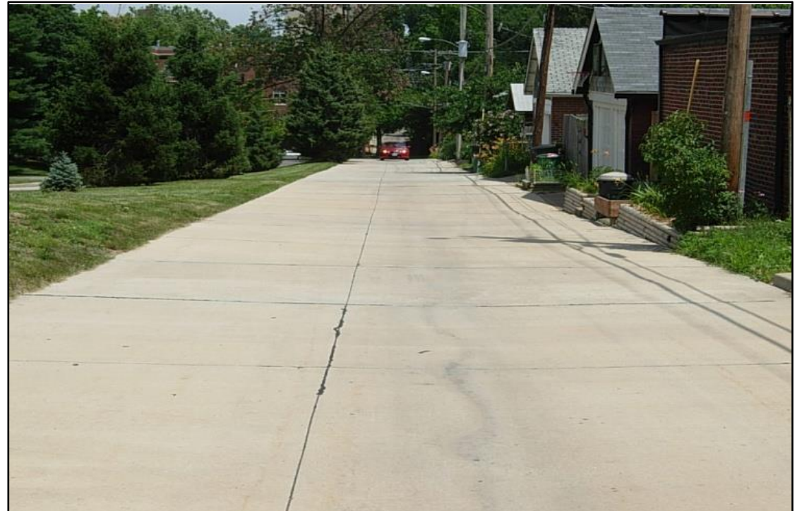
Project Location: Various Alleys 2019 and 2020.PW.1401.030
