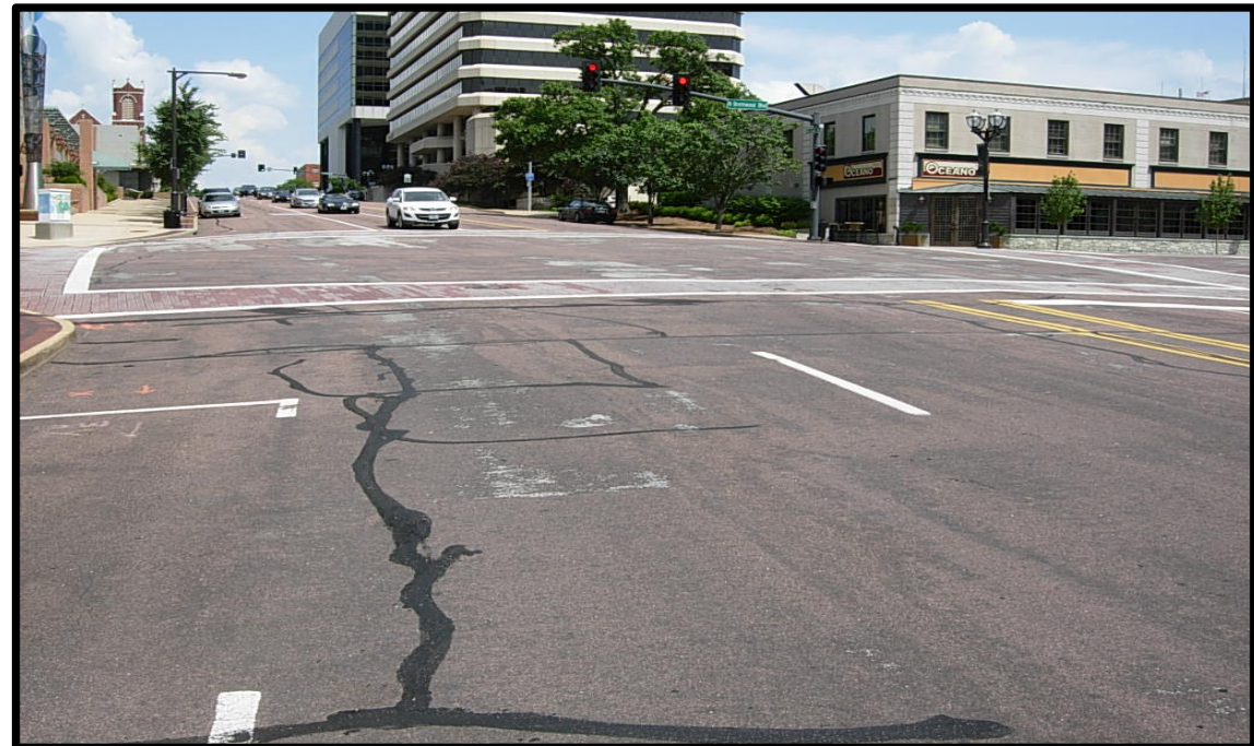
Project Location: Maryland Avenue BI.2019.PW.1401.011
