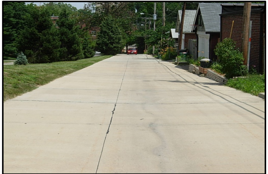
Project Location: Various Alleys 2019 and 2020.PW.1401.030
