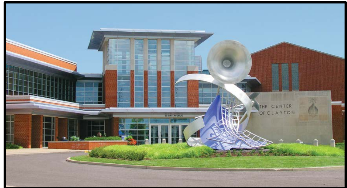
Project Location: The Center of Clayton
