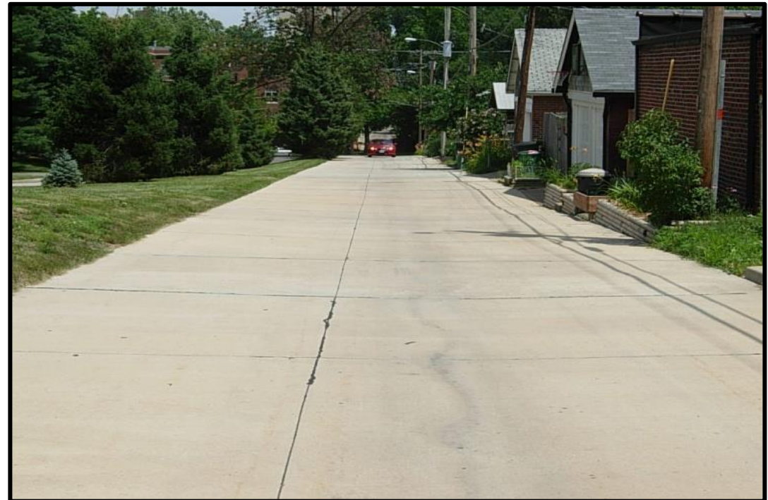
Project Location: Various Alleys 2019 and 2020.PW.1401.030
