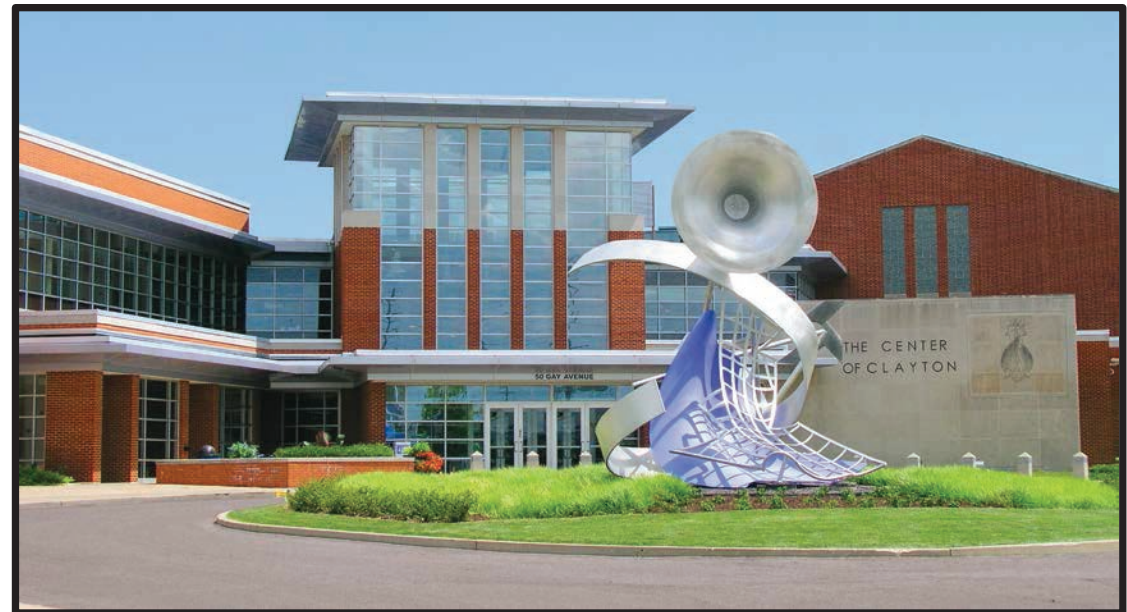
Project Location: The Center of Clayton
