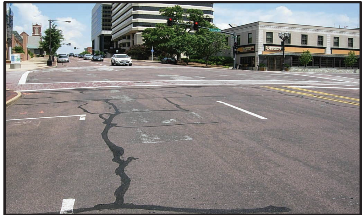
Project Location: Maryland Avenue BI.2019.PW.1401.011
