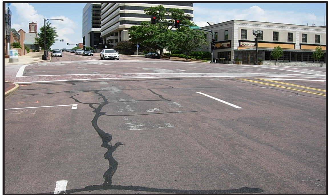
Project Location: Maryland Avenue BI.2019.PW.1401.011
