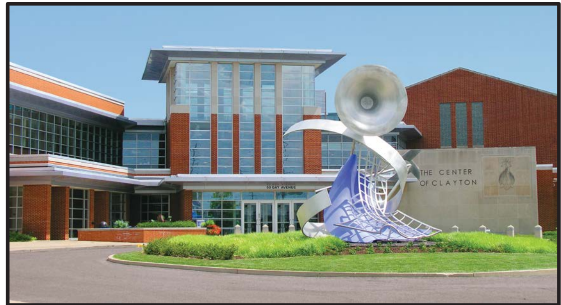
Project Location: The Center of Clayton
