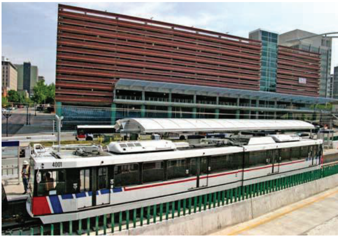
Shaw Park Drive Garage & Transit Center/ Clayton MetroBus Transfer Center
