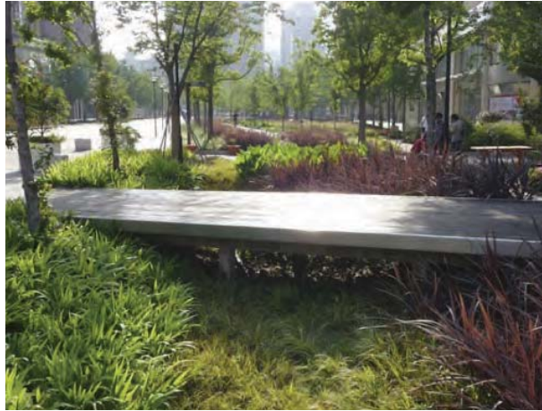
Pedestrian Bridge over Vegetated Swale
