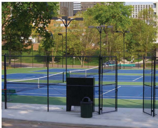
Existing Tennis Courts
