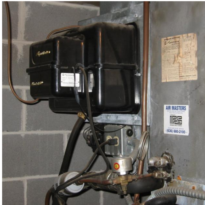
Mechanical (HVAC) Systems - Detail view to existing non-functioning humidifier unit [RIGHT].
