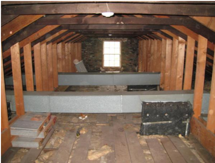
View to south showing existing attic conditions - seismic bracing would be recommended to provide additional loading surface for existing rafters at the tops of masonry walls.
