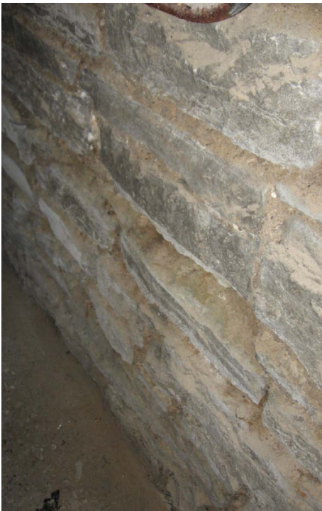
Interior Stone Masonry - Detail images depicting the condition of stone masonry foundation system, including settlement cracking at north wall [ABOVE LEFT], and view to masonry stair conditions at ground level cellar entry [RIGHT].
