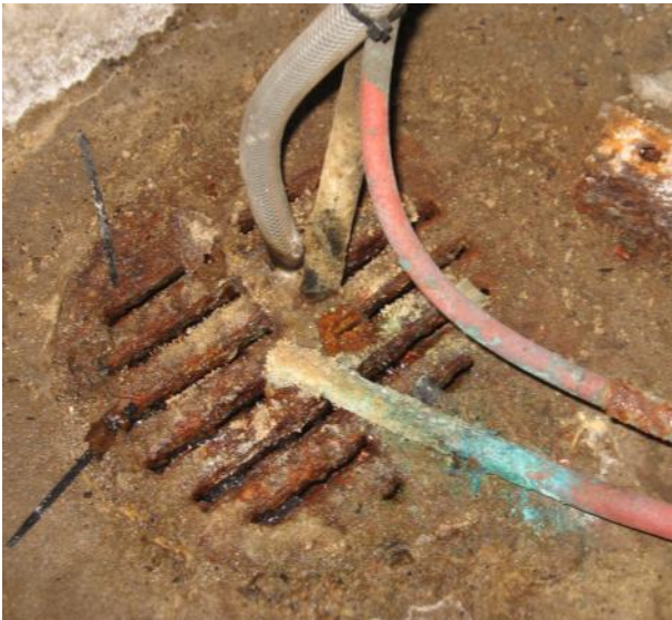
Mechanical (HVAC) Systems - Detail view to existing sheet metal combustion air ducting design [RIGHT] - this is likely to be considered a code violation if the Hanley House is significantly renovated and operated as a museum structure.
