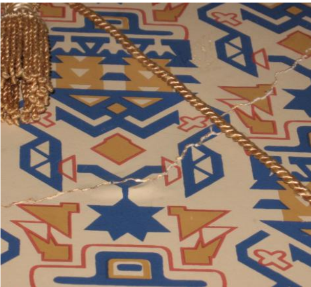
Detail image of interior plaster deterioration, including SW corner of Hanley House on face of flue adjacent to closet [ABOVE LEFT], and typical settlement cracking from corners of fenestration on first level [RIGHT].
