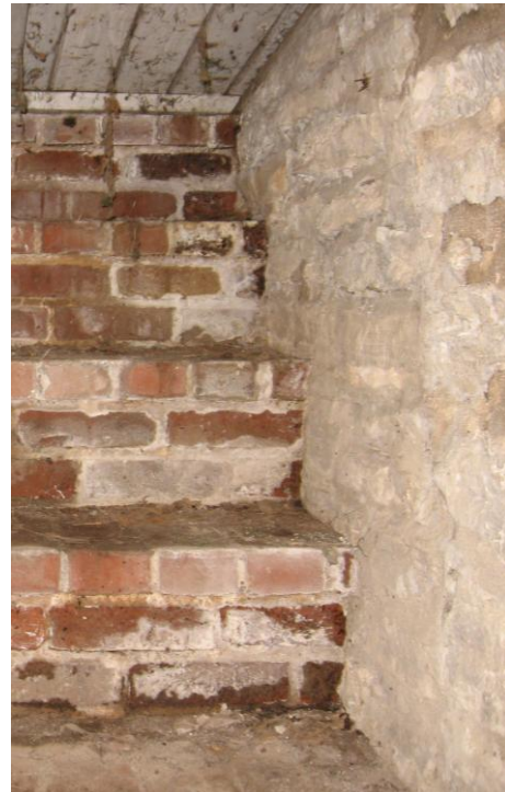
Interior Stone Masonry - Detail images depicting the condition of stone masonry foundation system, including settlement cracking at north wall [ABOVE LEFT], and view to masonry stair conditions at ground level cellar entry [RIGHT].
