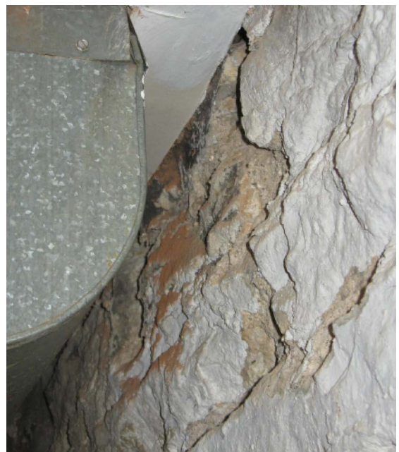
Interior Stone Masonry - Detail images depicting the condition of stone masonry foundation system, including settlement cracking at NE flue base and east wall [ABOVE LEFT and RIGHT].
