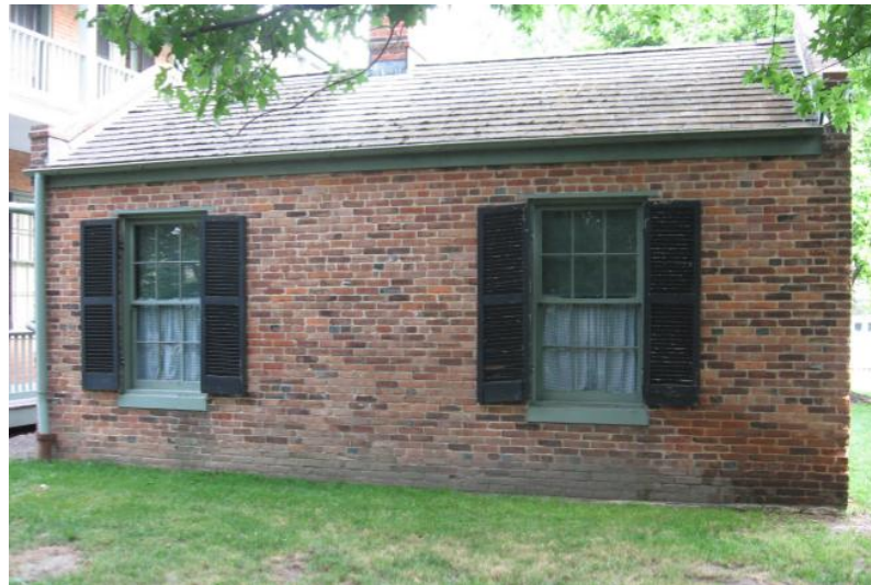
Exterior Windows and Wood Trim - Various images depicting wood shutters in need of repair at the Summer Kitchen.
