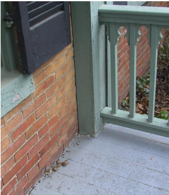
Exterior Wood Decks, Railings and Trim - Detail images depicting the condition of wood decking, trim, railings, and juncture to brick masonry at east two-level porch. At a minimum, this report would recommend the refurbishment of all wood carpentry items to include new finish.
