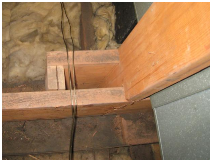
Roof Construction - Detail images show the existing roof system at attic level, including splice in typical double 2x12 beam running from north to south exterior bearing walls, and interior masonry conditions at attic level [TOP LEFT and ABOVE].
