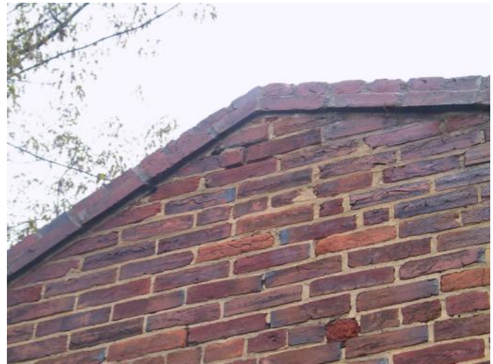
North Elevation Summer Kitchen - Above detail image shows deterioration of clay brick masonry due to impact from lawn sprinkler - masonry units are discolored and joints are failing. Detail image to left shows typical rotted wood cladding at eave and gutter.
