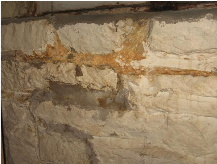
Interior Stone Masonry - Detail images depicting the condition of stone masonry foundation system, including settlement cracking at north wall [ABOVE LEFT], and view to masonry stair conditions at ground level cellar entry [RIGHT].
