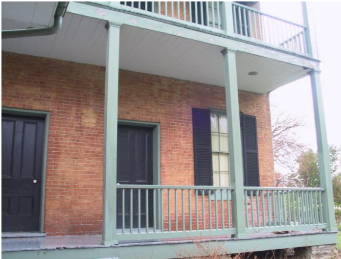
Exterior Wood Decks, Railings and Trim - Detail images depicting the condition of wood decking, trim, railings, and juncture to brick masonry at west two-level porch.
