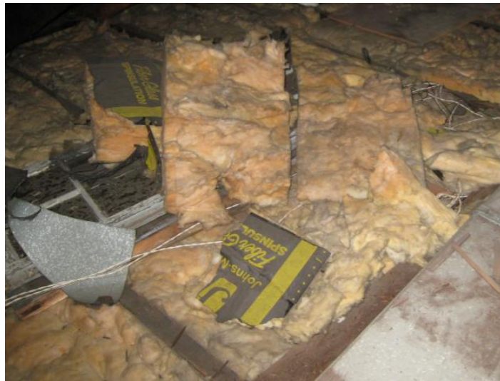
Detail images depicting condition of existing insulation in attic level floor joist spaces, sheet metal and other debris to be removed [LEFT and ABOVE] and supply air ducting design with partially insulated risers and main plumbing stack [BELOW RIGHT].
