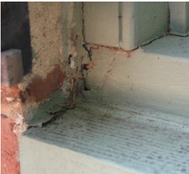
Summer Kitchen brick mould stops at subsill, which is strong evidence that these and possibly other windows throughout the Hanley House and Summer Kitchen were replaced during the ca. 1970 renovation scope.
