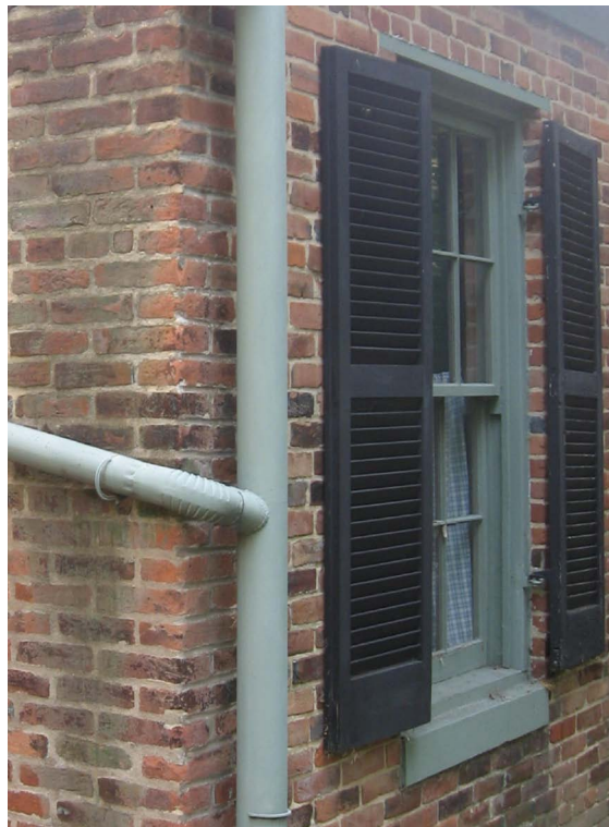
Summer Kitchen brick mould stops at subsill, which is strong evidence that these and possibly other windows throughout the Hanley House and Summer Kitchen were replaced during the ca. 1970 renovation scope.
