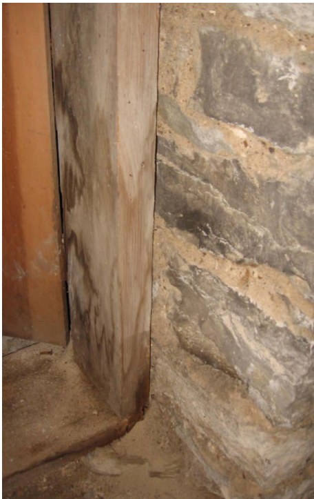
Detail images showing interior view to stone masonry foundation at south dirt floor area, including wood framing and trim members [RIGHT and BELOW RIGHT], and evidence of water infiltration through stone at west center door west jamb [BELOW LEFT].
