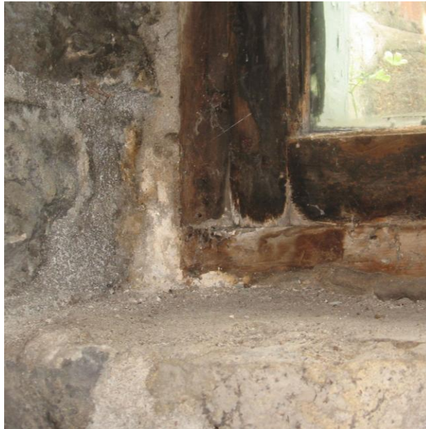
Detail images depicting the condition of first floor wood framing members off-set from stone masonry foundation system and bearing on steel clip angle [ABOVE LEFT], and typical clerestory window sash frame [ABOVE RIGHT] and stone masonry jamb and sill opening.
