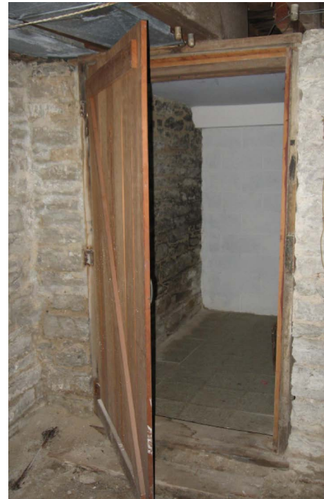
Detail images showing interior view to stone masonry foundation at south dirt floor area, including wood framing and trim members [RIGHT and BELOW RIGHT], and evidence of water infiltration through stone at west center door west jamb [BELOW LEFT].
