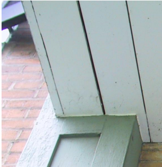
Exterior Wood Decks, Railings and Trim - Detail images depicting the condition of wood decking, trim, railings, and juncture to brick masonry at east two-level porch. At a minimum, this report would recommend the refurbishment of all wood carpentry items to include new finish.
