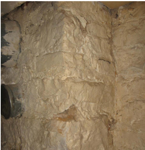
Interior Stone Masonry - Detail images depicting the condition of stone masonry foundation system, including settlement cracking at NE flue base and east wall [ABOVE LEFT and RIGHT].
