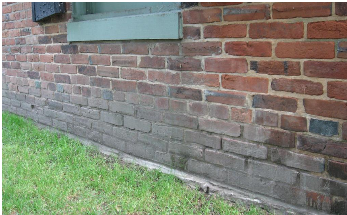
Brick existing conditions.
