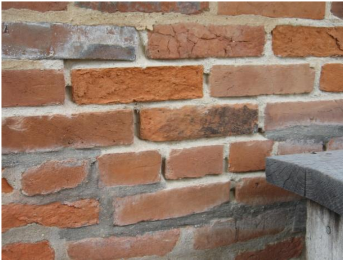
Brick existing conditions at Summer Kitchen.
