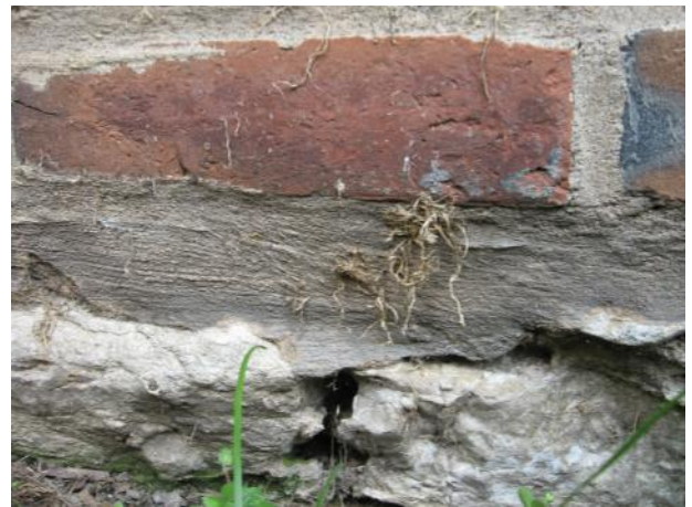
Stone foundation cracked and in need of repair.
