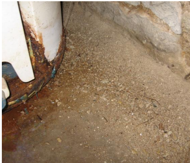
Existing ground level utility closet [ABOVE and LEFT] - note deteriorated domestic water heater and detritus on ground. The electric water heater has corroded through its tank, and is no longer serviceable.
