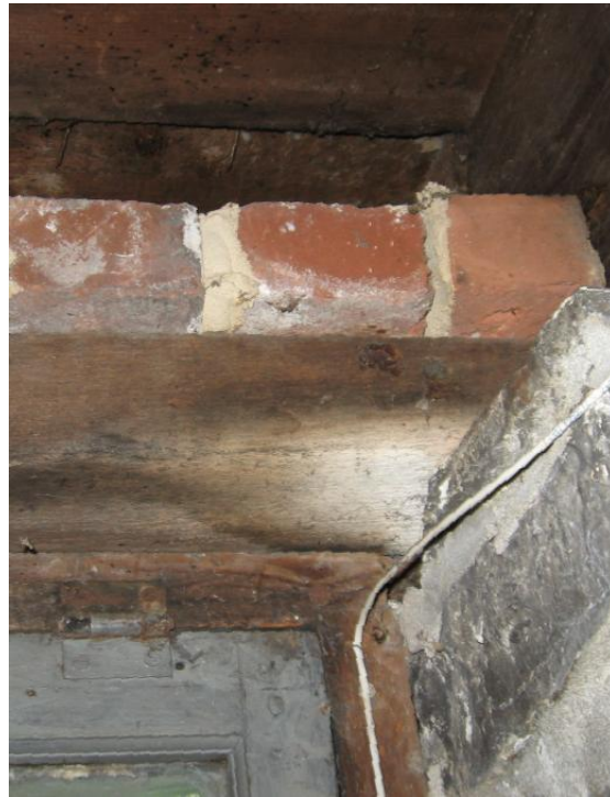
Interior Stone Masonry - Detail images depicting the condition of stone masonry foundation system, including head of west center door and lintel [ABOVE] to south dirt floor area, and at typical clerestory window head [RIGHT].
