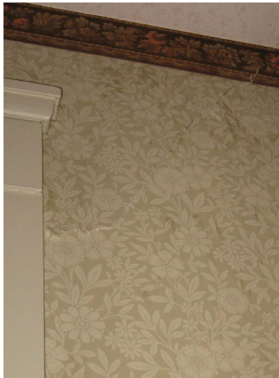
Detail image of interior plaster deterioration, including SW corner of Hanley House on face of flue adjacent to closet [ABOVE LEFT], and typical settlement cracking from corners of fenestration on first level [RIGHT].
