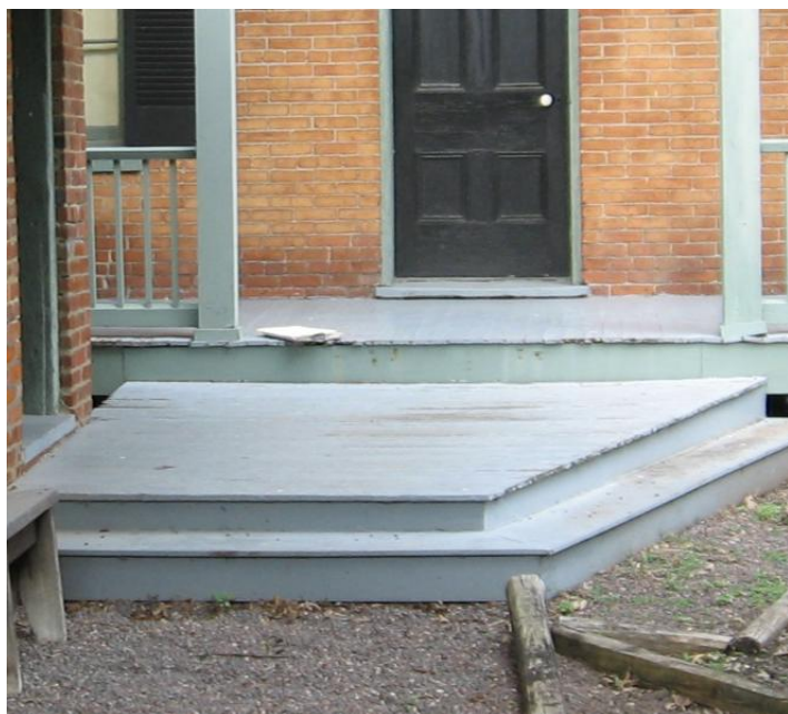
Exterior wood deck, existing conditions.
