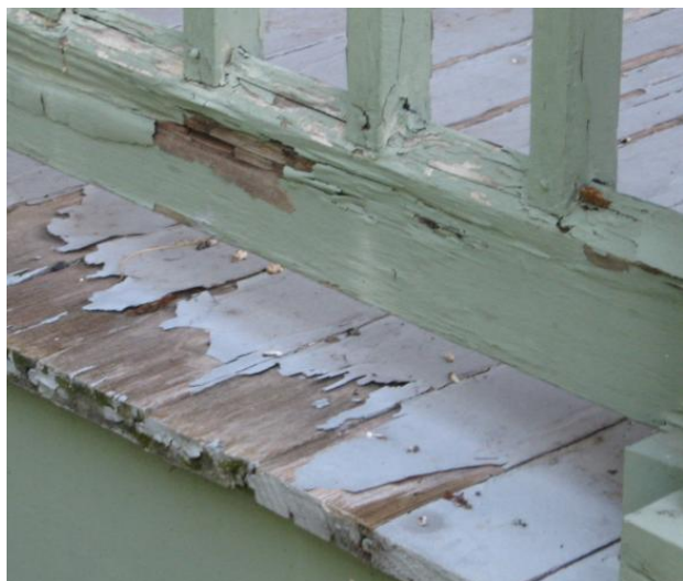
Detail images depicting the condition of wood decking, trim, railings, and juncture to brick masonry at west two-level porch. It is the understanding of this report that both the east and west porches were reconstructed ca. 1970.
