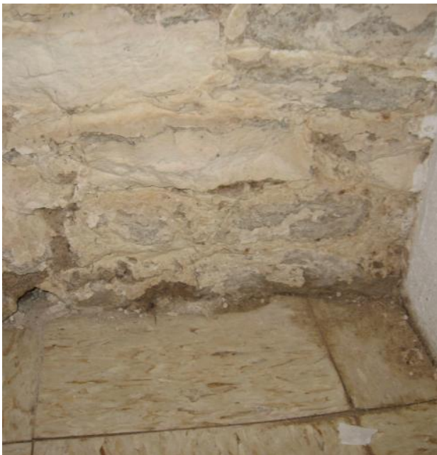
Existing ground level toilet [ABOVE LEFT and ABOVE RIGHT]. It appears that hydrostatic pressure has forced ground water through the stone foundation wall and up through the floor slab in this area. It is believed that the below-floor plumbing may no longer be serviceable.
