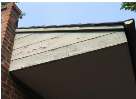
North Elevation Summer Kitchen - Above detail image shows deterioration of clay brick masonry due to impact from lawn sprinkler - masonry units are discolored and joints are failing. Detail image to left shows typical rotted wood cladding at eave and gutter.
