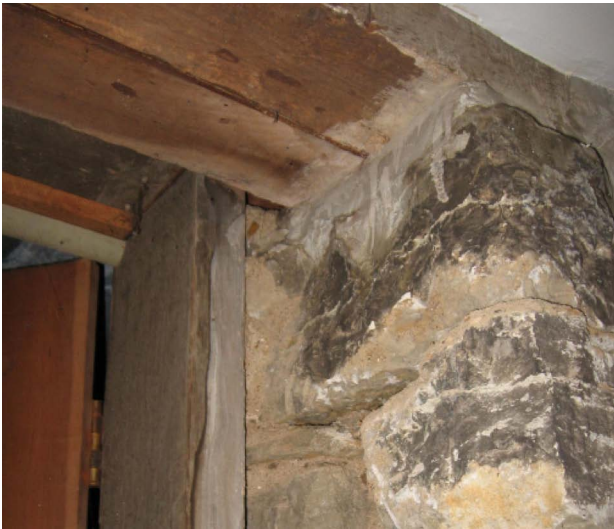
Interior Stone Masonry - Detail images depicting the condition of stone masonry foundation system, including head of west center door and lintel [ABOVE] to south dirt floor area, and at typical clerestory window head [RIGHT].
