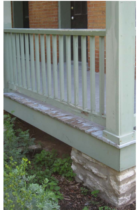
Exterior Wood Decks, Railings and Trim - Detail images depicting the condition of wood decking, trim, railings, and juncture to brick masonry at west two-level porch.
