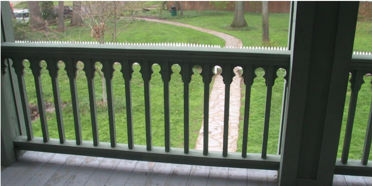
Exterior Wood Decks, Railings and Trim - Detail images depicting the condition of wood decking, trim, railings, and juncture to brick masonry at east two-level porch. At a minimum, this report would recommend the refurbishment of all wood carpentry items to include new finish.
