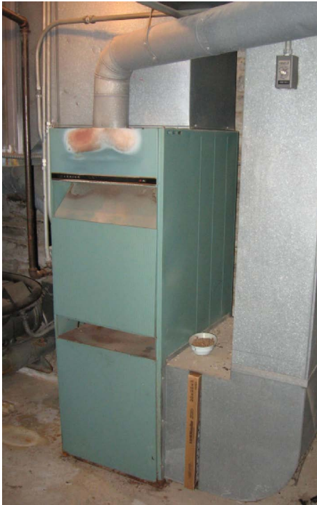
Detail views to typical existing furnace [LEFT] and water cooled condenser [ABOVE] units in ground level mechanical room, and existing typical floor drain in mechanical room [BELOW LEFT] for discharge of cooling water. These units are at the end of their serviceable life - it is the recommendation of this report that these units be replaced.
