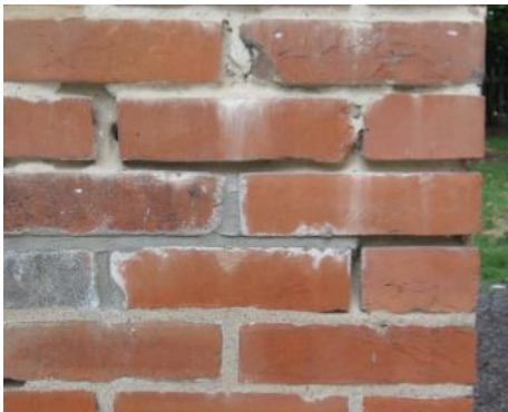
South Elevation Summer Kitchen - Detail image to right shows settlement crack at south end east parapet wall, while detail image below shows typical failed mortar joints at middle SE corner.
