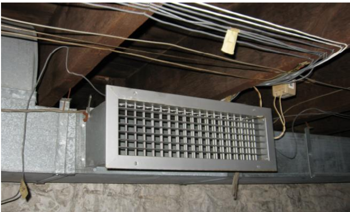
Existing duct routing.
