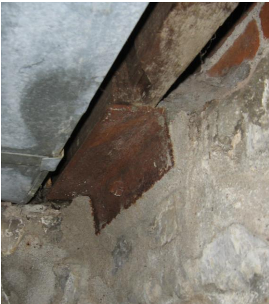
Detail images depicting the condition of first floor wood framing members off-set from stone masonry foundation system and bearing on steel clip angle [ABOVE LEFT], and typical clerestory window sash frame [ABOVE RIGHT] and stone masonry jamb and sill opening.
