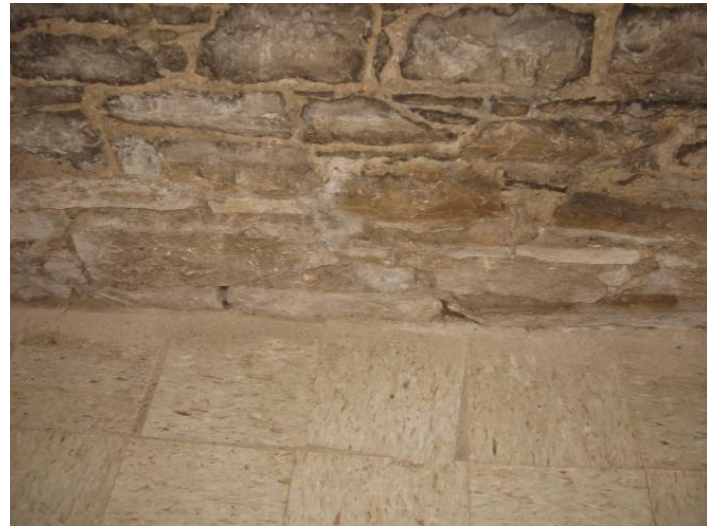
Interior stone masonry wall conditions at the central corridor in the home's lower level suggest that hydrostatic pressure has forced ground water through the stone foundation walls (original) and concrete floor slab (ca. 1969) in this area.
