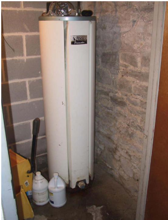
Existing ground level utility closet [ABOVE and LEFT] - note deteriorated domestic water heater and detritus on ground. The electric water heater has corroded through its tank, and is no longer serviceable.
