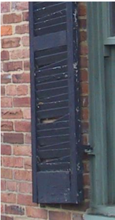
Exterior Windows and Wood Trim - Various images depicting wood shutters in need of repair at the Summer Kitchen.
