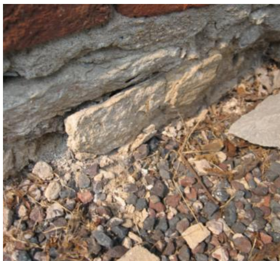
Stone foundation existing conditions.
