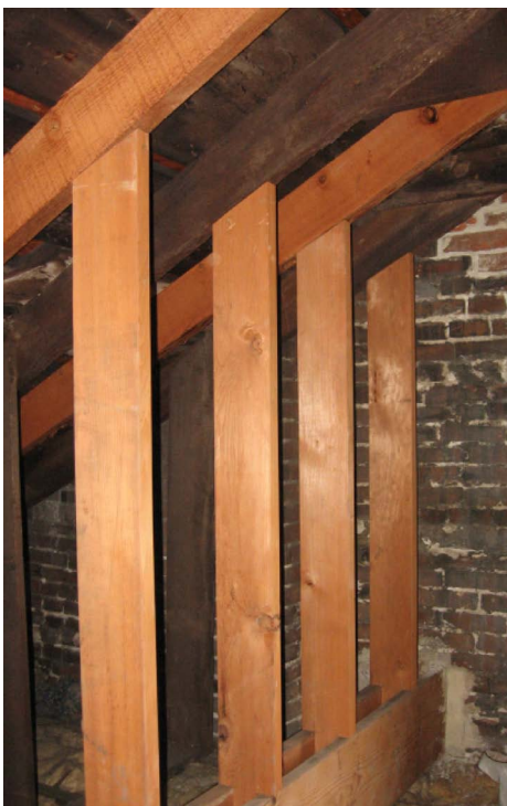
Roof Construction - Detail images show the existing roof system at attic level, including splice in typical double 2x12 beam running from north to south exterior bearing walls, and interior masonry conditions at attic level [TOP LEFT and ABOVE].
