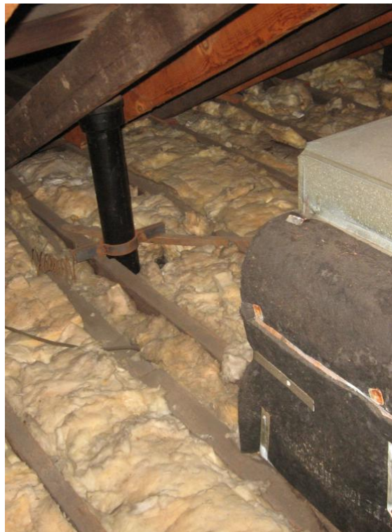
Detail image of obstructed roof hatch from attic level interior - hatch was likely concealed during ca. 1970 renovation work, and would be recommended for re-opening to perform future maintenance and / or roof replacement work.
