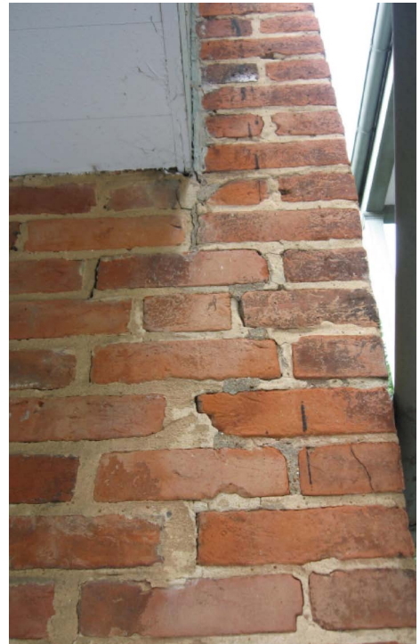
South Elevation Summer Kitchen - Detail image to right shows settlement crack at south end east parapet wall, while detail image below shows typical failed mortar joints at middle SE corner.
