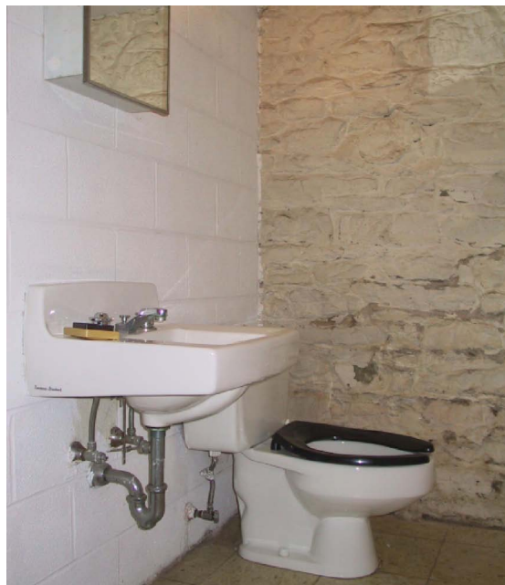
Existing ground level toilet [ABOVE LEFT and ABOVE RIGHT]. It appears that hydrostatic pressure has forced ground water through the stone foundation wall and up through the floor slab in this area. It is believed that the below-floor plumbing may no longer be serviceable.
