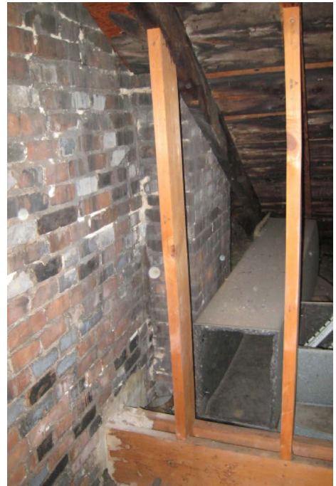
View to south showing existing attic conditions - seismic bracing would be recommended to provide additional loading surface for existing rafters at the tops of masonry walls.
