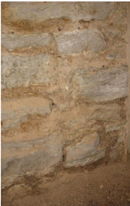
Interior stone masonry wall conditions at the central corridor in the home's lower level suggest that hydrostatic pressure has forced ground water through the stone foundation walls (original) and concrete floor slab (ca. 1969) in this area.
