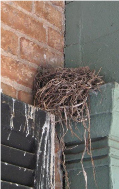
Detail view to typical cornice, column cap and trim area that would be recommended for anti-bird devices to be installed [LEFT].
