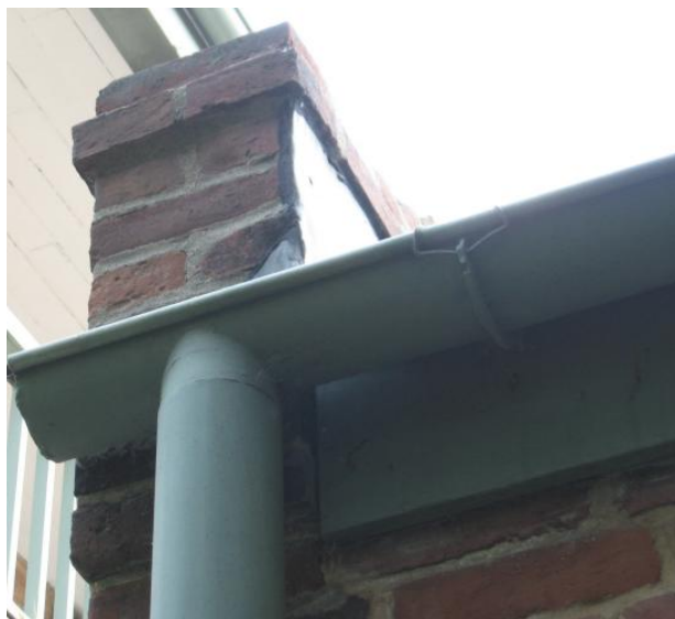
Existing gutter system and downspouts.
