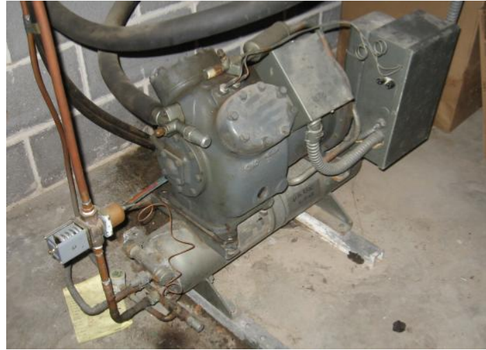
Detail views to typical existing furnace [LEFT] and water cooled condenser [ABOVE] units in ground level mechanical room, and existing typical floor drain in mechanical room [BELOW LEFT] for discharge of cooling water. These units are at the end of their serviceable life - it is the recommendation of this report that these units be replaced.
