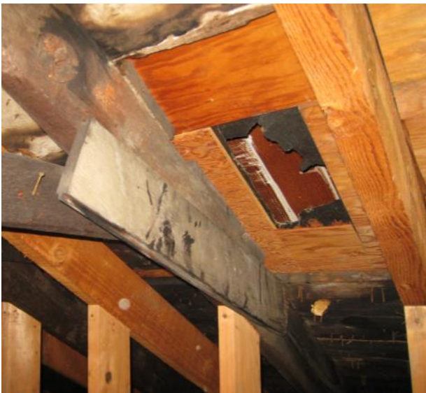
Detail image of obstructed roof hatch from attic level interior - hatch was likely concealed during ca. 1970 renovation work, and would be recommended for re-opening to perform future maintenance and / or roof replacement work.
