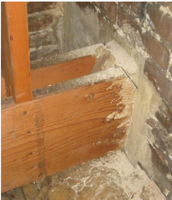
Roof Construction - Detail images show the existing roof system at the attic level, including typical double 2x12 beam running from north to south exterior bearing walls [BOTTOM LEFT], and interior masonry conditions at attic level [BOTTOM RIGHT].
