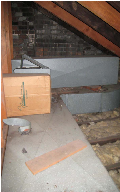
Detail images depicting condition of existing insulation in attic level floor joist spaces, sheet metal and other debris to be removed [LEFT and ABOVE] and supply air ducting design with partially insulated risers and main plumbing stack [BELOW RIGHT].
