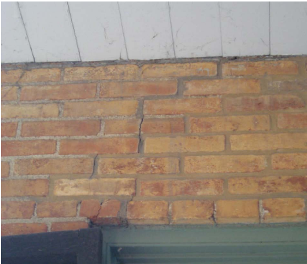
Exterior Clay Brick Masonry - Detail images depicting the condition of west facing clay brick masonry, including below roof overhang at attic level west porch [ABOVE], and at SW corner [RIGHT] where some tuckpointing has been done.
