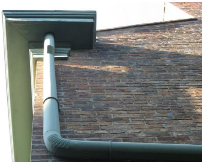
Sheet Metal Gutter and Downspouts - Detail images show routing of downspouts from box gutter (at Hanley House east) toward Summer Kitchen and termination at storm water boots and below-grade storm sewerage. Hung gutters [BELOW] are shallow but appear to be adequately sized.
