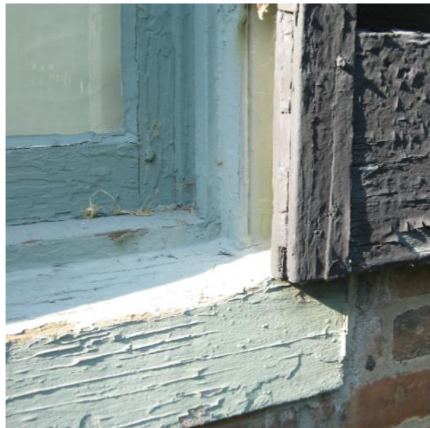
Detail images show typical conditions of sash, sill and shutter at first level north [ABOVE LEFT and RIGHT]. These sills are not clad like the south elevation sills, but their finish is failed and the likelihood of moisture having contributed to deterioration of the window units is high. Note design of trim end is scalloped - this flourish is typical at all north (and south equal) elevation sills.
