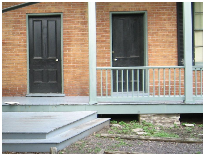
View to doors at first level west elevation [ABOVE] Detail image of typical exterior wood door condition [LEFT], showing original hardware, and failed finish on raised panel, stile-and-rail construction wood slab.
