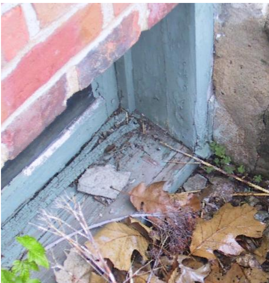
Exterior Wood Windows - Detail images show condition of typical clerestory units at Hanley House ground level [ABOVE LEFT and RIGHT]. Wood sills, jambs, and window sash frames appear to be rotten, with finishes failed and in need of replacement. Note that unpainted steel lintels were installed - possibly ca. 1970 - at the SW and both north clerestory openings. These lintels are serviceable, but are recommended to be ground and painted.
