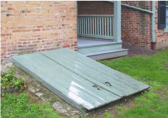
Detail view to ground level entry through wood cellar doors [ABOVE], at NW corner of Hanley House. Note relatively shallow depth of porch, between west wall and railing [ABOVE and RIGHT]. With the addition of a ramp, these west doors and porch represent a potential secondary egress route to grade, if the structure is classified as a commercial occupancy for the sake of renovations.
