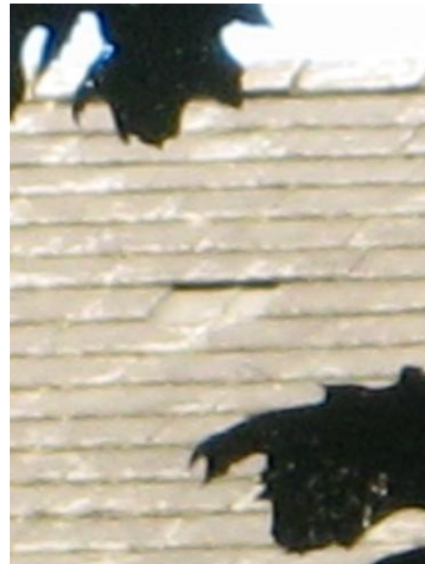
Roof Construction - Detail image to right shows missing cement roof tile at east facing field. Moss is visible in several areas of east facing roof, as are oddly spaced roof tiles.
