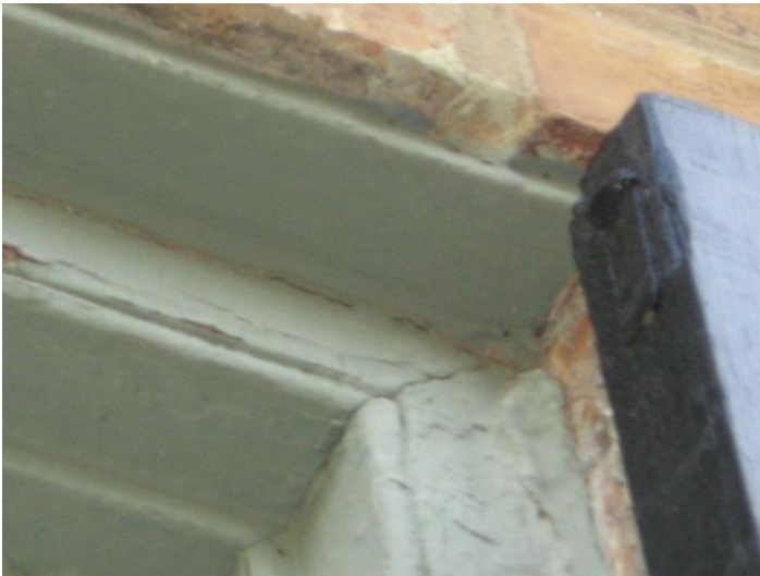
Exterior Wood Windows - Detail images show designs and conditions of various Hanley House lintels, including painted steel angle at first level south [ABOVE], and no apparent lintel with brick row-lock header at first level north [RIGHT]. Steel angle lintels do not appear to be original.
