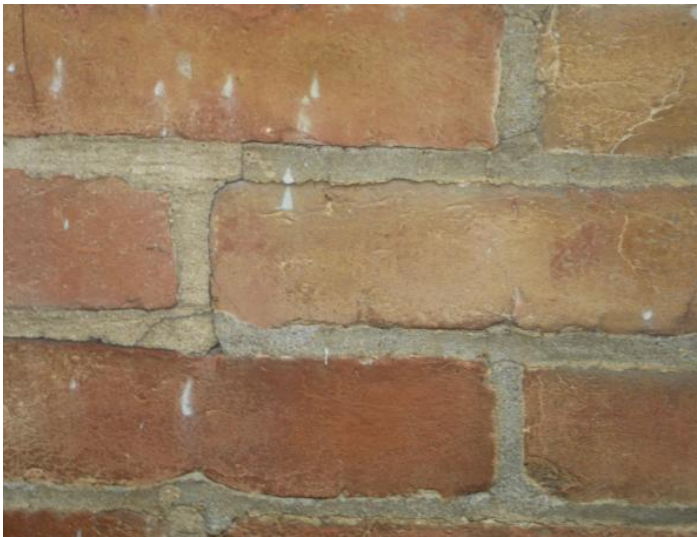
Detail view to typical east facing clay brick masonry [ABOVE and LEFT], showing deteriorated and non-serviceable mortar conditions. Note that replacement mortar appears to have been installed in shallow depths, and in varying colors, hardnesses, and joint dimensions.
