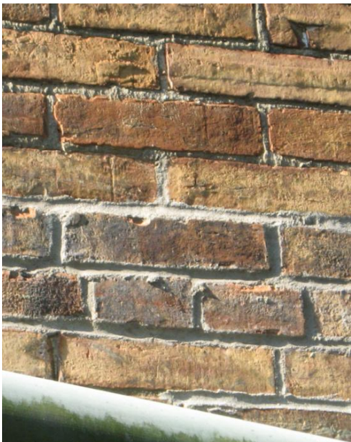
Detail image [ABOVE RIGHT] depicts degree to which ca. 1970 renovations are expected to have addressed deteriorated clay brick above first level window heads at north.
