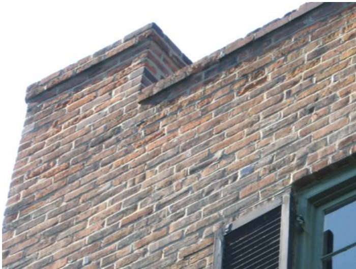
Exterior Clay Brick Masonry - Detail images depict the conditions of high points clay brick masonry at Hanley House north including north, west [ABOVE], east and south [RIGHT] faces of NE chimney. Note the appearance of brick units with spalled or pocked faces - these may be interior wythe brick which were original to the house, but which were relocated to the building exterior as a repair.
