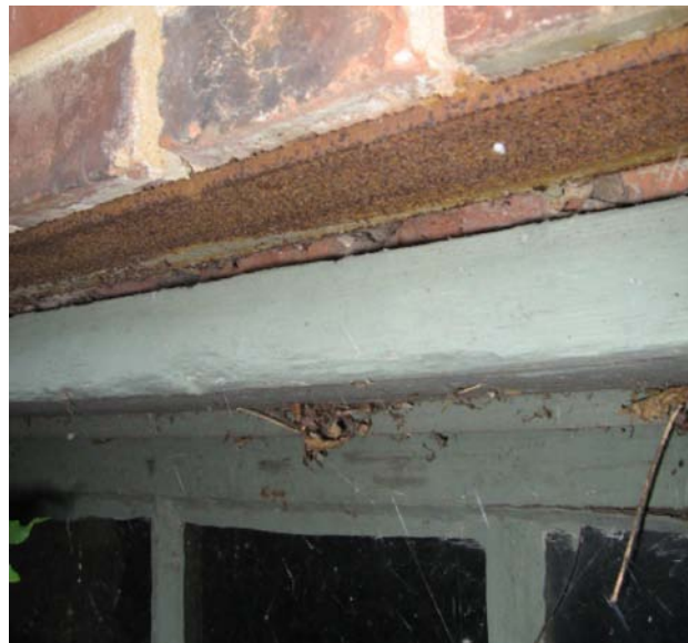
Exterior Wood Windows - Detail images show condition of typical clerestory units at Hanley House ground level [ABOVE LEFT and RIGHT]. Wood sills, jambs, and window sash frames appear to be rotten, with finishes failed and in need of replacement. Note that unpainted steel lintels were installed - possibly ca. 1970 - at the SW and both north clerestory openings. These lintels are serviceable, but are recommended to be ground and painted.
