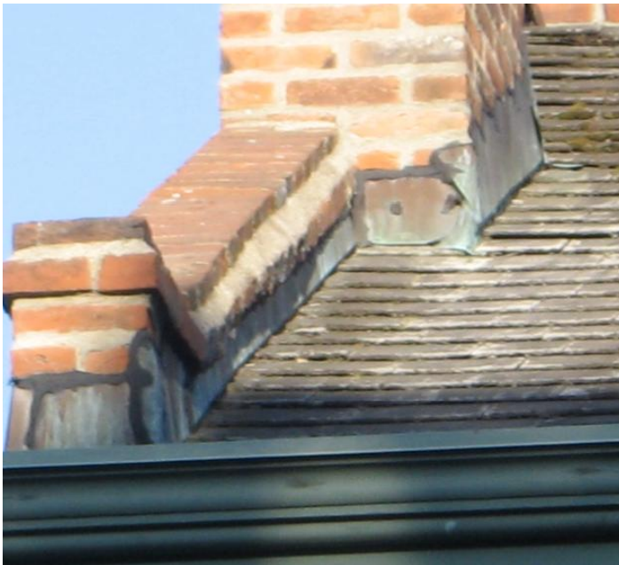
Roof Construction - Detail image to right shows missing cement roof tile at east facing field. Moss is visible in several areas of east facing roof, as are oddly spaced roof tiles.
