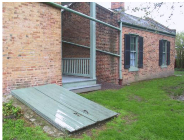
Summer Kitchen North Elevation
