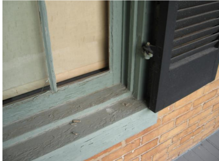
Exterior Wood Windows, Decks, Railings and Trim - Detail images depict various deteriorated conditions of windows and surrounding original trim at Hanley House, including typical window fenestration design at first level east under porch [LEFT], and typical sash and sill at second level west under porch [ABOVE].
