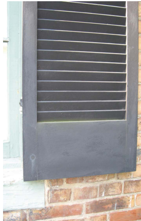
Exterior Wood Shutters - Detail images show various conditions of existing Hanley House shutters, including original position-holding hardware [ABOVE], typical replacement shutter [RIGHT], and extreme component and finish deterioration encountered on original shutters.
