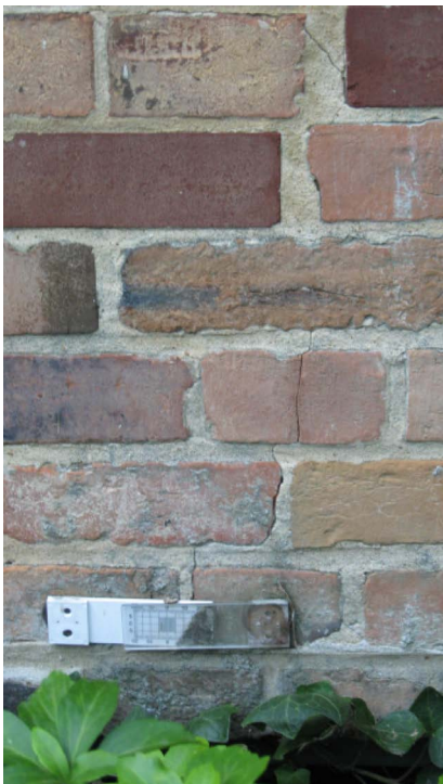
View to North Elevation [ABOVE] Detail view to east most settlement crack at north [LEFT]
