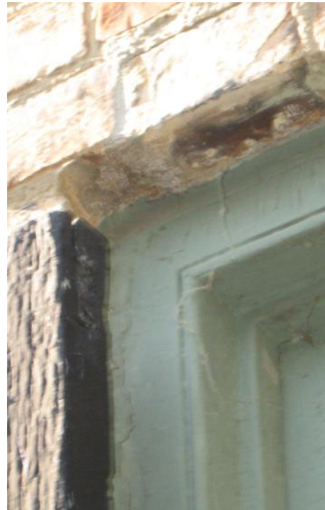
Exterior Wood Windows - Detail images show designs and conditions of various Hanley House lintels, including painted steel angle at first level south [ABOVE], and no apparent lintel with brick row-lock header at first level north [RIGHT]. Steel angle lintels do not appear to be original.
