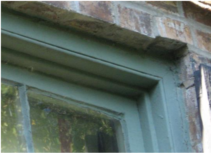
Exterior Wood Windows - Detail image shows design and condition of no apparent lintel with brick row-lock header at first level north [ABOVE] Hanley House. Note that brick header is off-set and bowed downward due to a lack of structural capacity - the brick above this typical opening is likely supported entirely by the wood window unit.
