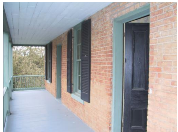
View to North at West Porch Second Level
