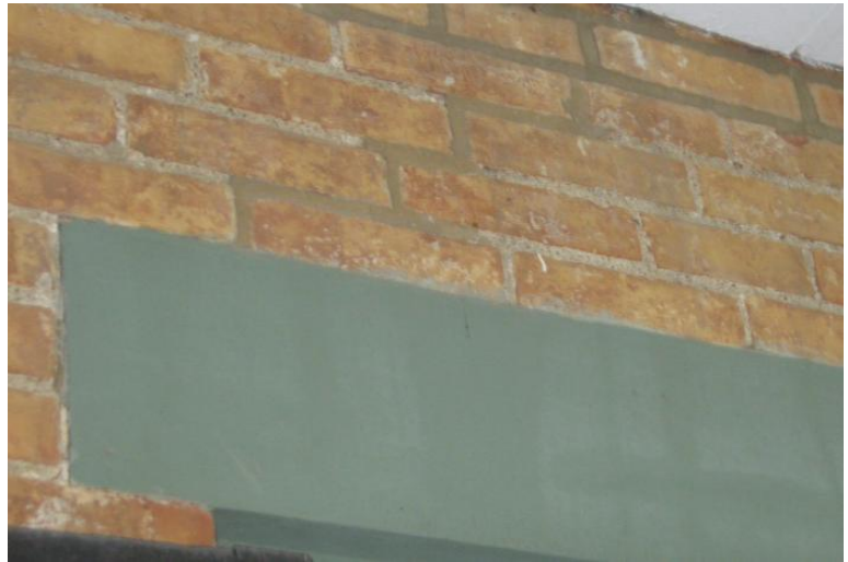
Exterior Clay Brick Masonry - Detail images depict the conditions of east facing clay brick masonry, including patch replacement brick [LEFT], settlement cracks below first level fenestration at wood timber lintel [TOP RIGHT], field joint failure at tuckpointed mortar [BOTTOM LEFT], and settlement cracking at NE corner below first level fenestration [BOTTOM RIGHT].
