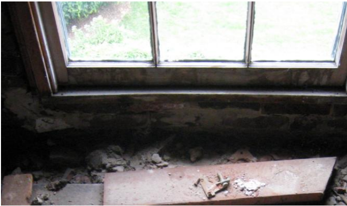
Exterior Wood Windows - Detail images show typical condition of window units and trim at Hanley House attic level [ABOVE and RIGHT]. Wood sills, jambs, and window sash frames appear to be rotten, with finishes failed and in need of replacement. Evidence in the attic at both north and south ends suggest that original glass panes were re-glazed into replacement sashes - possibly ca. 1970. Also, there are glazed shutters abandoned in the attic which may once have been employed to vent and close the attic at each end.
