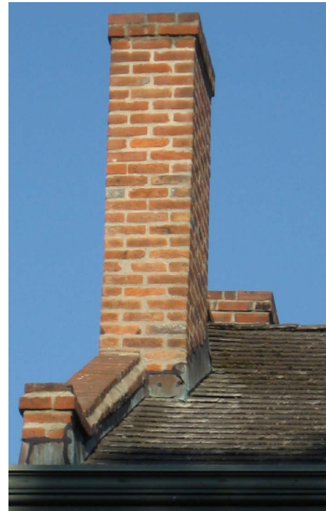
Roof Construction - East elevation [LEFT] shows orientation of roof pitch with box gutter and gable design. Detail images to right and below depict typical relationship between masonry bearing walls, projected parapets, chimneys (four such), sheet metal flashings, and cement tile finish roof. Note arrangement of low parapet wall as termination for roof system.
