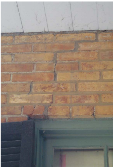
Exterior Wood Windows - Detail images show no apparent lintel with brick row-lock header at first level west [ABOVE LEFT], and painted wood timber at first level east [ABOVE RIGHT]. Although wood timber lintels (found only at the east elevation of Hanley House) appear to be original, they are at the end of serviceable life. This report would recommend that all windows not already supported by one be augmented by a concealed steel angle - said steel could be installed behind the exterior wythe of clay brick, and could be painted to match. All steel should be flashed to evacuate water.
