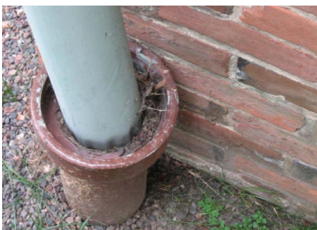
Drainage of storm water from the Hanley House and Summer Kitchen roofs is compounded not only by the lengthy, twisted routing from initial collection to final sewerage, but also by the quantity of disposal. It is presumed that historic authenticity directed only 2 such storm water boots [LEFT]
