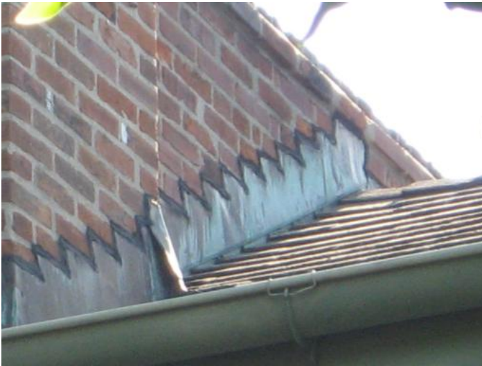
Roof Construction - Detail images show sheet metal step flashing to parapet walls and sealant joints [TOP LEFT], clay masonry parapet end-of-wall condition and wood trim [TOP RIGHT], typical roof hatch in west-facing roof field [BOTTOM RIGHT], and wood trim at box gutter with sheet metal pipe downspout. Note that hatch is covered and not accessible from interior at attic level.
