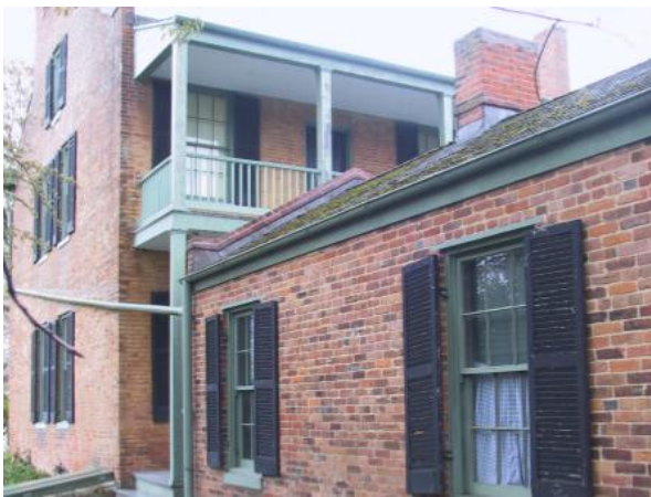
Partial Hanley House West Elevation [LEFT]
