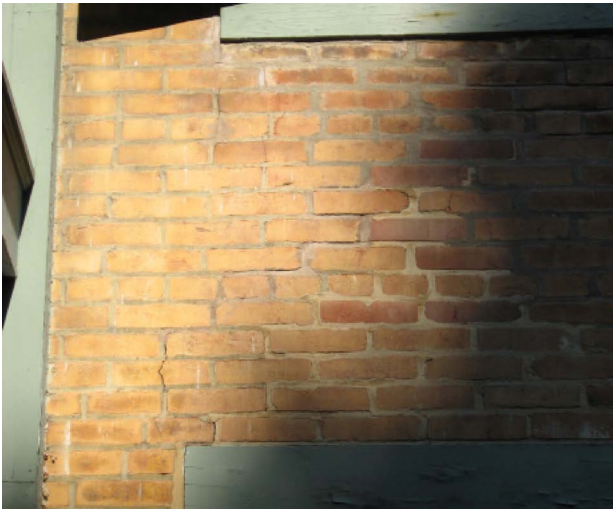
Exterior Clay Brick Masonry - Detail views to east facing clay brick masonry showing settlement cracking at north fenestration, first and second levels. Note that mortar joints and brick units have cracked through at north extent of east elevation immediately above foundation [BELOW LEFT].
