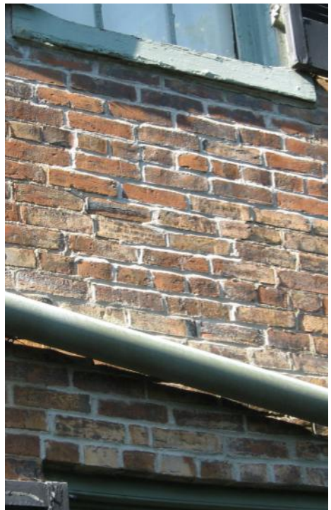
Detail images showing limited tuckpointing repair at brick masonry field [ABOVE] and between first and second level fenestration on north side [RIGHT].
