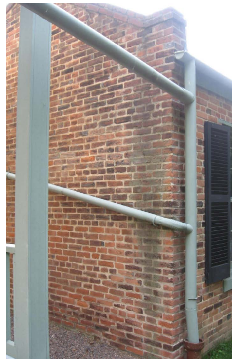
Sheet Metal Gutter and Downspouts - Detail images show routing of downspouts from box gutter (at Hanley House east) toward Summer Kitchen and termination at storm water boots and below-grade storm sewerage. Hung gutters [BELOW] are shallow but appear to be adequately sized.
