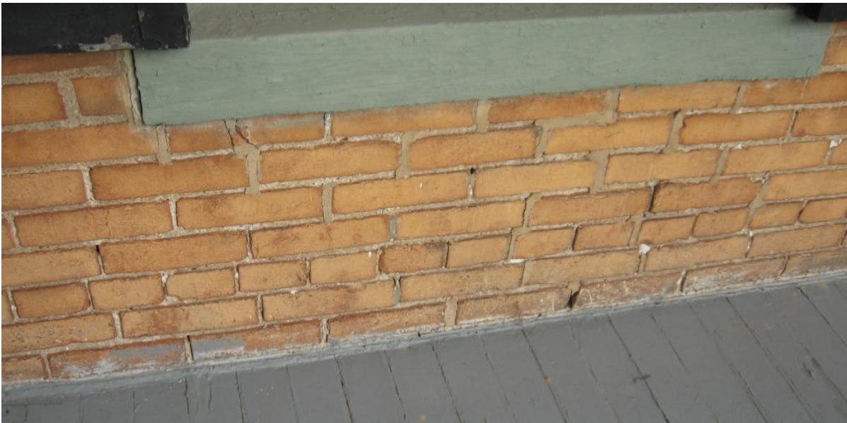
Detail image depicting the condition of west facing clay brick masonry immediately above first level west porch floor [above]. Note quantity of open, failed, and missing mortar joints below window sill. Despite protection provided by the west porch overhang, this area demonstrates continued movement and deterioration of exterior clay brick masonry, and should be repaired.
