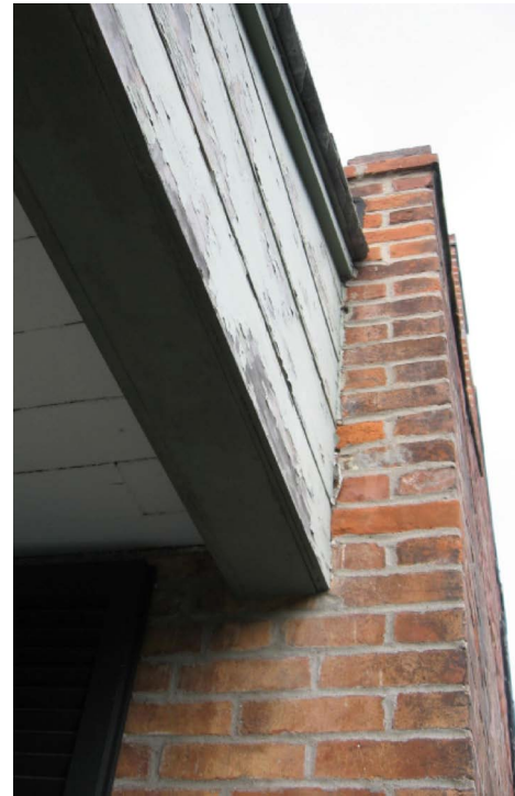
Roof Construction - Detail images show sheet metal step flashing to parapet walls and sealant joints [TOP LEFT], clay masonry parapet end-of-wall condition and wood trim [TOP RIGHT], typical roof hatch in west-facing roof field [BOTTOM RIGHT], and wood trim at box gutter with sheet metal pipe downspout. Note that hatch is covered and not accessible from interior at attic level.
