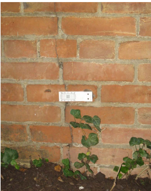
Detail view to east facing settlement crack in clay brick masonry [ABOVE LEFT], showing abandoned crack monitor device. Note that tuckpointed mortar joints at some areas of the east have been installed in a tooled (canted) profile - this is different than virtually all other (flush) joints.
