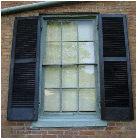
Exterior Wood Windows - Views to various Hanley House window conditions showing original and replaced sashes and glazing. Images include second level west fenestration and trim under porch [TOP LEFT], attic level north fenestration and trim [ABOVE RIGHT], and first level south fenestration and trim [ABOVE LEFT]. Note that all items in these views appear to be original except the sash frame at attic level north (with south being equal); glazing in these sash frames may be original.
