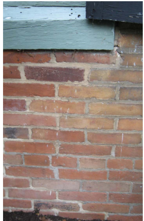
Detail view to typical east facing clay brick masonry [ABOVE and LEFT], showing deteriorated and non-serviceable mortar conditions. Note that replacement mortar appears to have been installed in shallow depths, and in varying colors, hardnesses, and joint dimensions.
