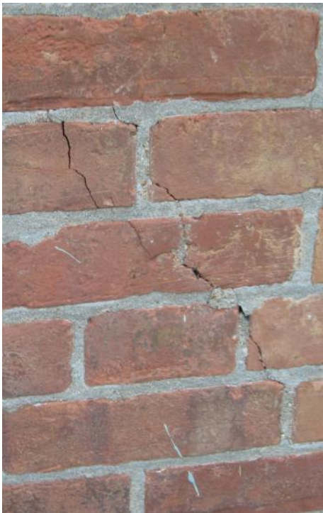
Exterior Clay Brick Masonry - Detail images depict the conditions of south facing clay brick masonry, including settlement cracks below first level fenestration [TOP LEFT and RIGHT], and long-run settlement cracking at SW corner [BOTTOM LEFT and RIGHT], extending from near stone foundation upward to parapet and SW chimney.
