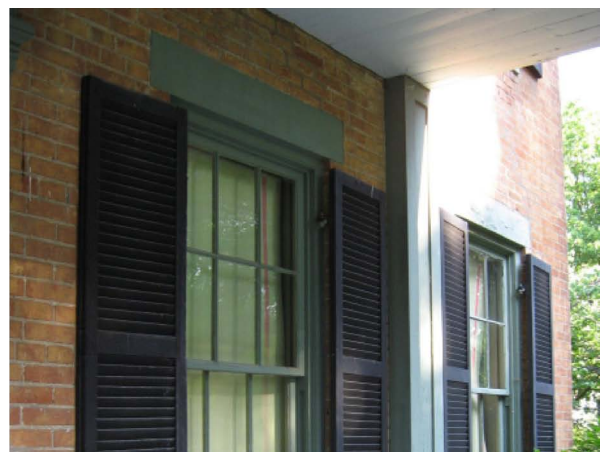
Typical East-Facing Windows
