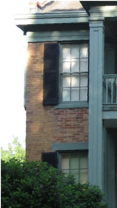
Exterior Clay Brick Masonry - Detail images depict the conditions of east facing clay brick masonry, including patch replacement brick [LEFT], settlement cracks below first level fenestration at wood timber lintel [TOP RIGHT], field joint failure at tuckpointed mortar [BOTTOM LEFT], and settlement cracking at NE corner below first level fenestration [BOTTOM RIGHT].
