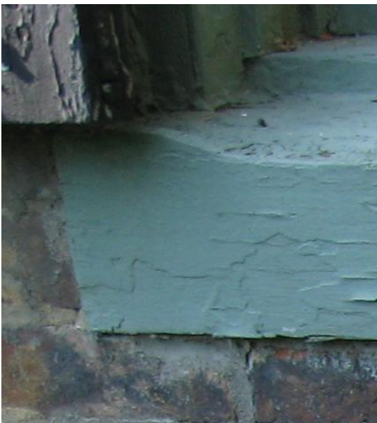
Detail images show typical conditions of sash, sill and shutter at first level north [ABOVE LEFT and RIGHT]. These sills are not clad like the south elevation sills, but their finish is failed and the likelihood of moisture having contributed to deterioration of the window units is high. Note design of trim end is scalloped - this flourish is typical at all north (and south equal) elevation sills.
