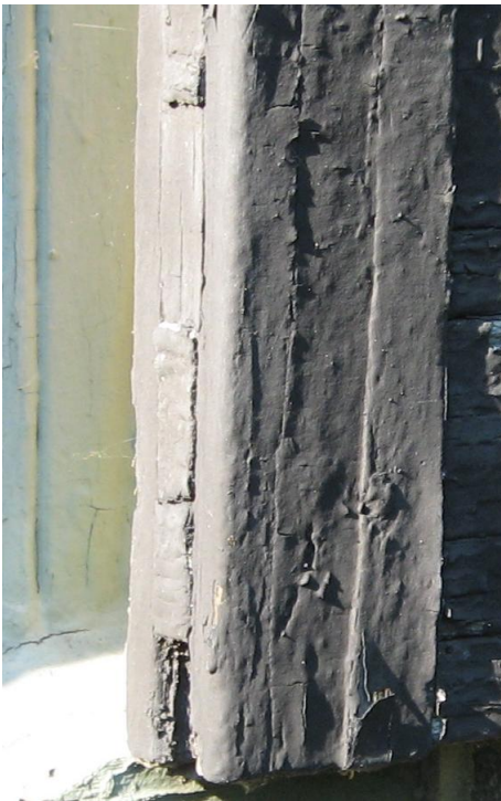
Exterior Wood Shutters - Detail images show various conditions of existing Hanley House shutters, including original position-holding hardware [ABOVE], typical replacement shutter [RIGHT], and extreme component and finish deterioration encountered on original shutters.
