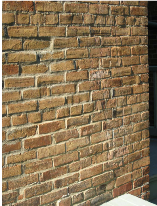
Detail images showing limited tuckpointing repair at brick masonry field [ABOVE and BELOW] and above wood cellar doors on north side [RIGHT].
