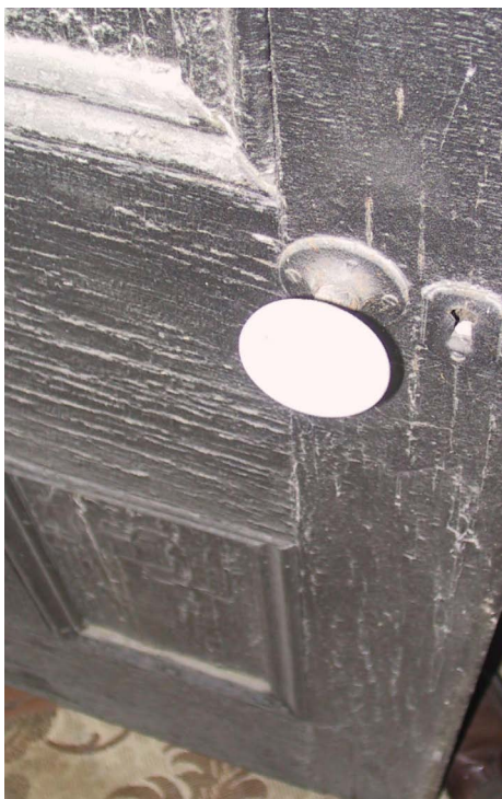
View to doors at first level west elevation [ABOVE] Detail image of typical exterior wood door condition [LEFT], showing original hardware, and failed finish on raised panel, stile-and-rail construction wood slab.
