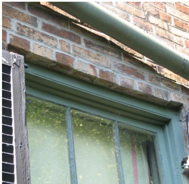
Detail image [ABOVE RIGHT] depicts degree to which ca. 1970 renovations are expected to have addressed deteriorated clay brick above first level window heads at north.
