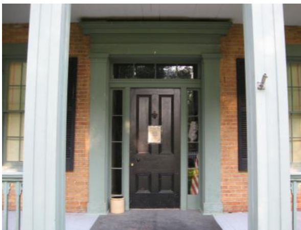
View to Main Entry at East Porch [LEFT]
