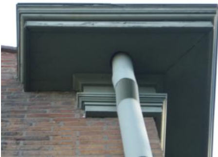
Roof Construction - Detail images show sheet metal step flashing to parapet walls and sealant joints [TOP LEFT], clay masonry parapet end-of-wall condition and wood trim [TOP RIGHT], typical roof hatch in west-facing roof field [BOTTOM RIGHT], and wood trim at box gutter with sheet metal pipe downspout. Note that hatch is covered and not accessible from interior at attic level.
