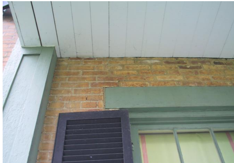
Exterior Wood Windows - Detail images show no apparent lintel with brick row-lock header at first level west [ABOVE LEFT], and painted wood timber at first level east [ABOVE RIGHT]. Although wood timber lintels (found only at the east elevation of Hanley House) appear to be original, they are at the end of serviceable life. This report would recommend that all windows not already supported by one be augmented by a concealed steel angle - said steel could be installed behind the exterior wythe of clay brick, and could be painted to match. All steel should be flashed to evacuate water.
