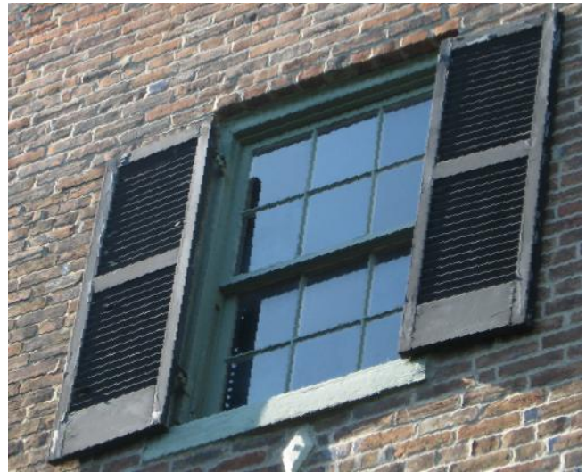
Exterior Wood Windows - Views to various Hanley House window conditions showing original and replaced sashes and glazing. Images include second level west fenestration and trim under porch [TOP LEFT], attic level north fenestration and trim [ABOVE RIGHT], and first level south fenestration and trim [ABOVE LEFT]. Note that all items in these views appear to be original except the sash frame at attic level north (with south being equal); glazing in these sash frames may be original.
