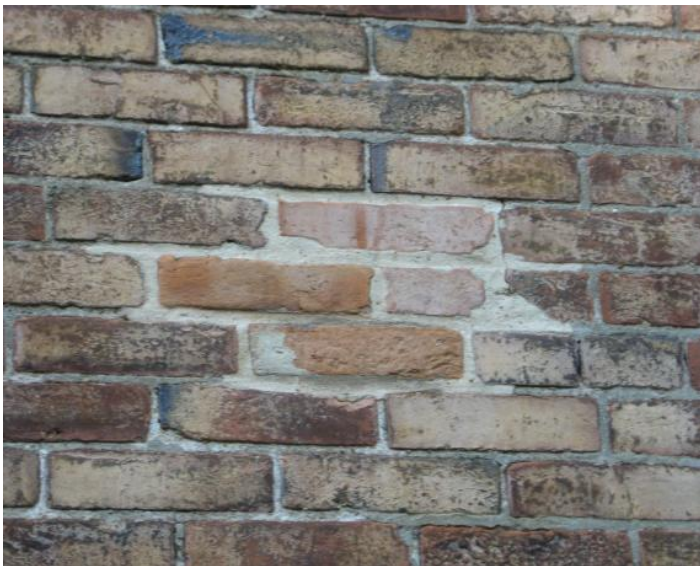
Detail images showing limited tuckpointing repair at brick masonry field [ABOVE] and between first and second level fenestration on north side [RIGHT].
