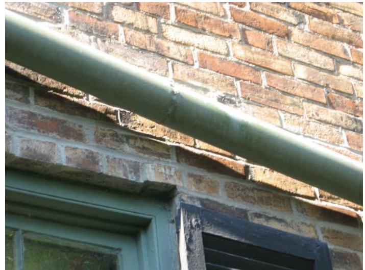
Drainage of storm water from the Hanley House and Summer Kitchen roofs is compounded not only by the lengthy, twisted routing from initial collection to final sewerage, but also by the quantity of disposal. It is presumed that historic authenticity directed only 2 such storm water boots [LEFT]
