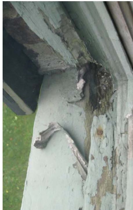
Exterior Wood Windows - Detail images show typical condition of window units and trim at Hanley House attic level [ABOVE and RIGHT]. Wood sills, jambs, and window sash frames appear to be rotten, with finishes failed and in need of replacement. Evidence in the attic at both north and south ends suggest that original glass panes were re-glazed into replacement sashes - possibly ca. 1970. Also, there are glazed shutters abandoned in the attic which may once have been employed to vent and close the attic at each end.
