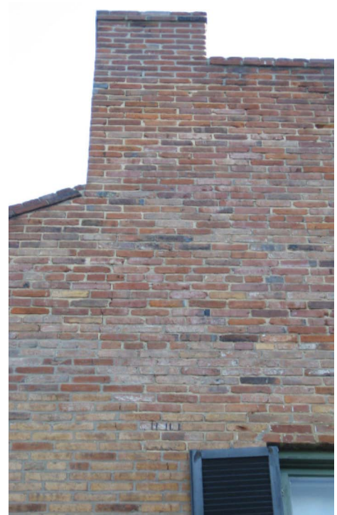
Exterior Clay Brick Masonry - Detail images depict the relationship of attic level fenestration and chimneys at partial north elevation [TOP LEFT], and long-run settlement cracking at SW chimney [RIGHT].
