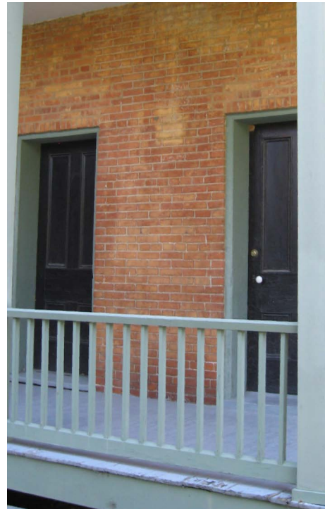
Detail view to ground level entry through wood cellar doors [ABOVE], at NW corner of Hanley House. Note relatively shallow depth of porch, between west wall and railing [ABOVE and RIGHT]. With the addition of a ramp, these west doors and porch represent a potential secondary egress route to grade, if the structure is classified as a commercial occupancy for the sake of renovations.
