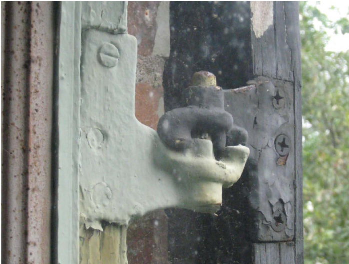
Exterior Wood Shutters - Detail images show various conditions of existing Hanley House shutters, including original position-holding hardware [ABOVE], typical replacement shutter [RIGHT], and extreme component and finish deterioration encountered on original shutters.
