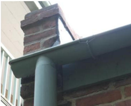
Sheet Metal Gutter and Downspouts - Detail images show routing of downspouts from box gutter (at Hanley House east) toward Summer Kitchen and termination at storm water boots and below-grade storm sewerage. Hung gutters [BELOW] are shallow but appear to be adequately sized.
