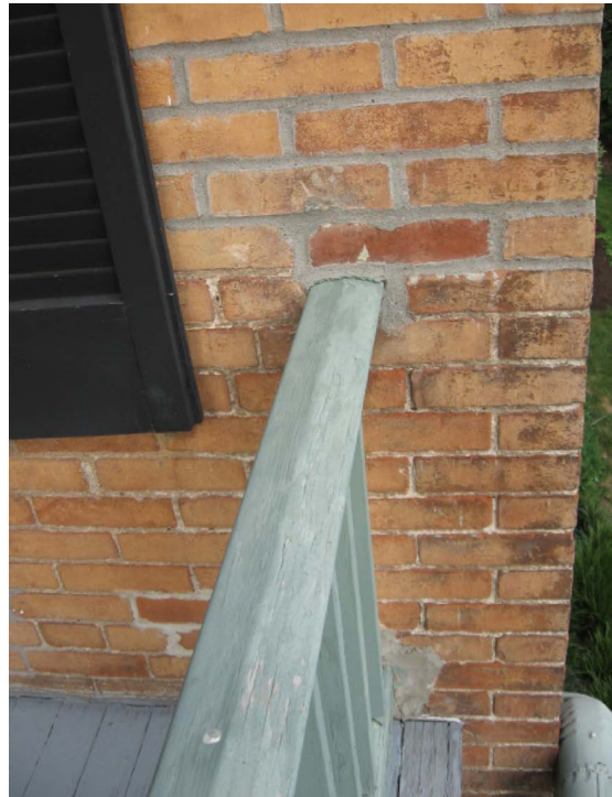
Exterior Clay Brick Masonry - Detail images depicting the condition of west facing clay brick masonry, including below roof overhang at attic level west porch [ABOVE], and at SW corner [RIGHT] where some tuckpointing has been done.
