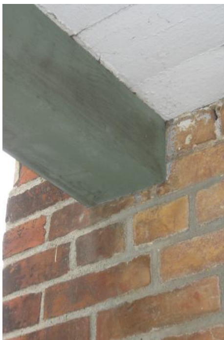
Exterior Clay Brick Masonry - Detail images depict the conditions of high points clay brick masonry at Hanley House north including north, west [ABOVE], east and south [RIGHT] faces of NE chimney. Note the appearance of brick units with spalled or pocked faces - these may be interior wythe brick which were original to the house, but which were relocated to the building exterior as a repair.
