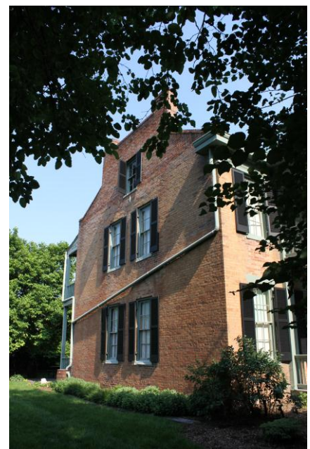
FIGURE G-2, Hanley House exterior
