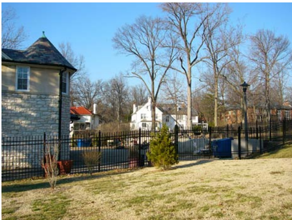
OAK KNOLL PARK , Maintenance Facility Yard
