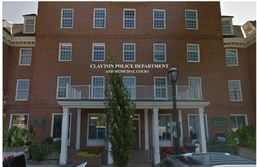
Project Location: 10 S. Brentwood Blvd 2020.PW.40.42.442
