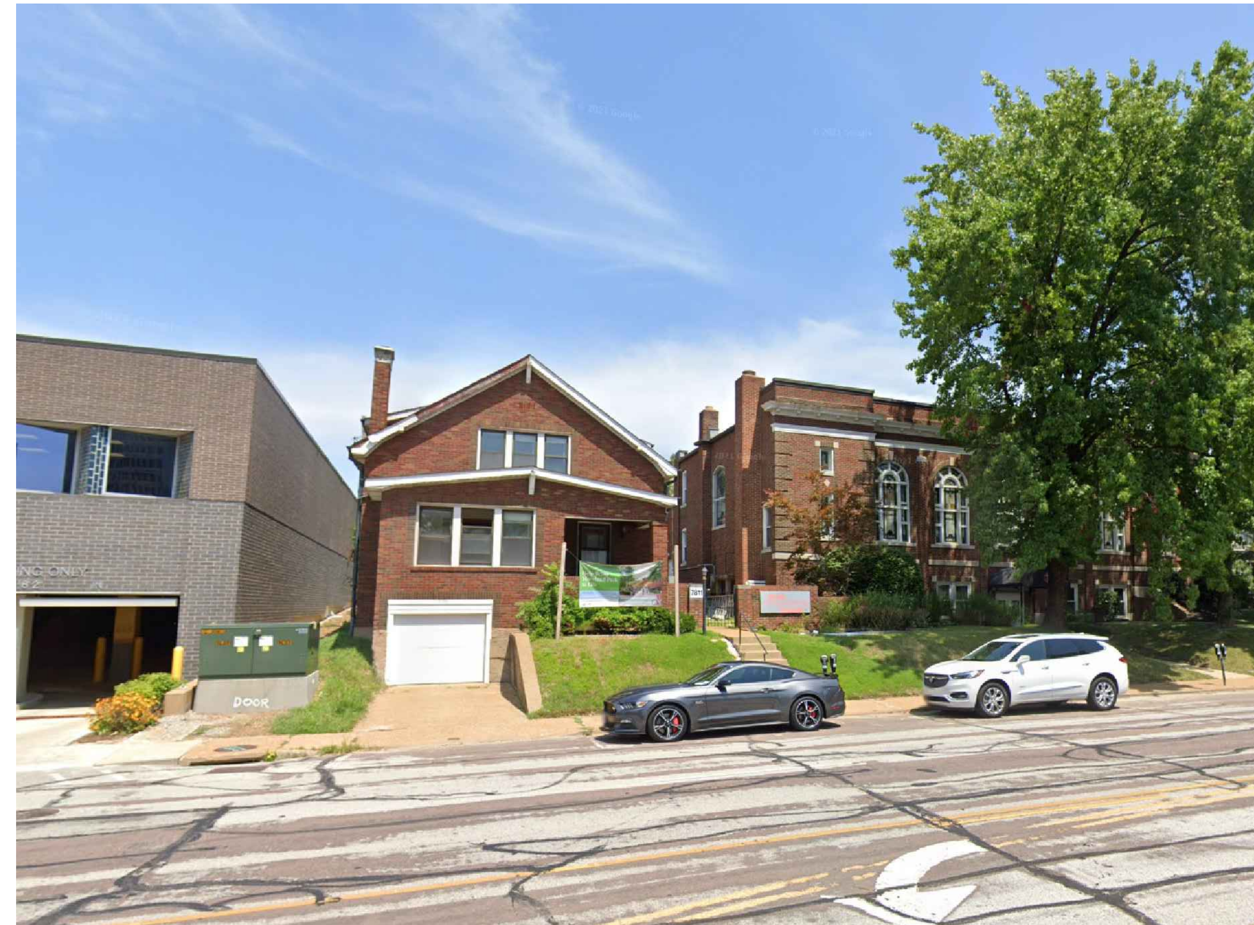
EXISTING SITE PHOTO
